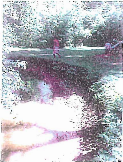
Photo 16: Eroded pool in ROW north of Chattman
