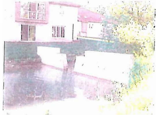
Photo 4: Example of alternate spillway configuration (Macomb Township, MI)
