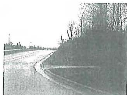
Significant vegetation removal would be required with centerline road widening.
