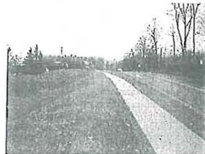
Looking east, road widening will cause slope challenges behind sidewalk.
