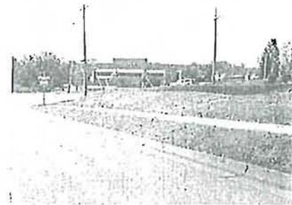
Widening of the road will result in relocation of narrow greenbelt and adjacent sidewalk.
