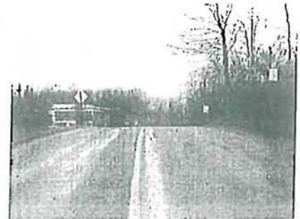
A site distance analysis may reveal crest vertical curve concerns on a green signal phase.
