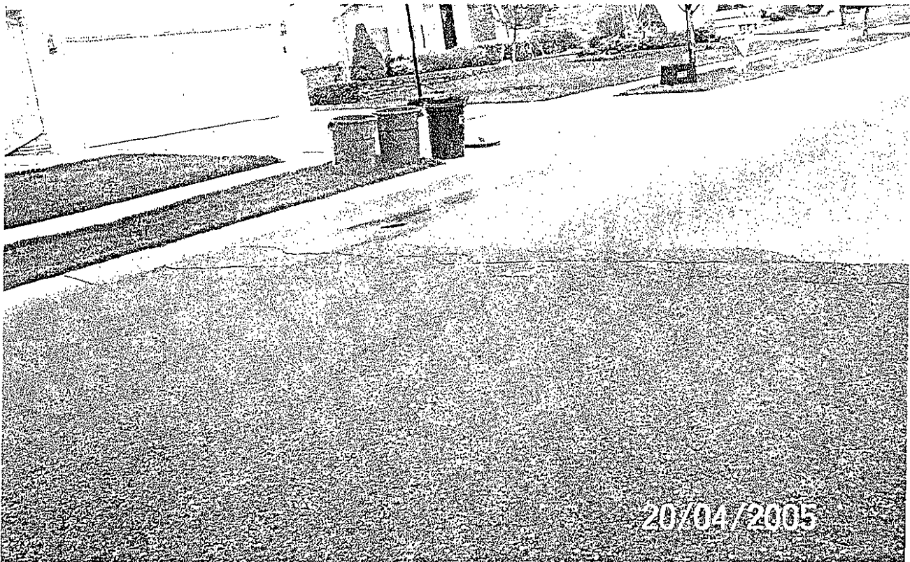
Sandstone at house no. 43116 Typical transverse cracking. Occurs frequently on this street at intervals of 100 ft. +/-
