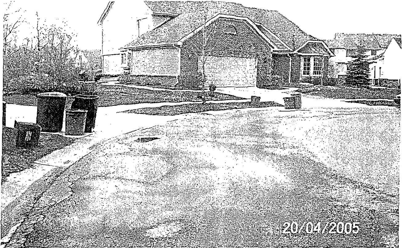
Ledgeview at house no. 42745 Ponding near edge of metal and edge cracking.
