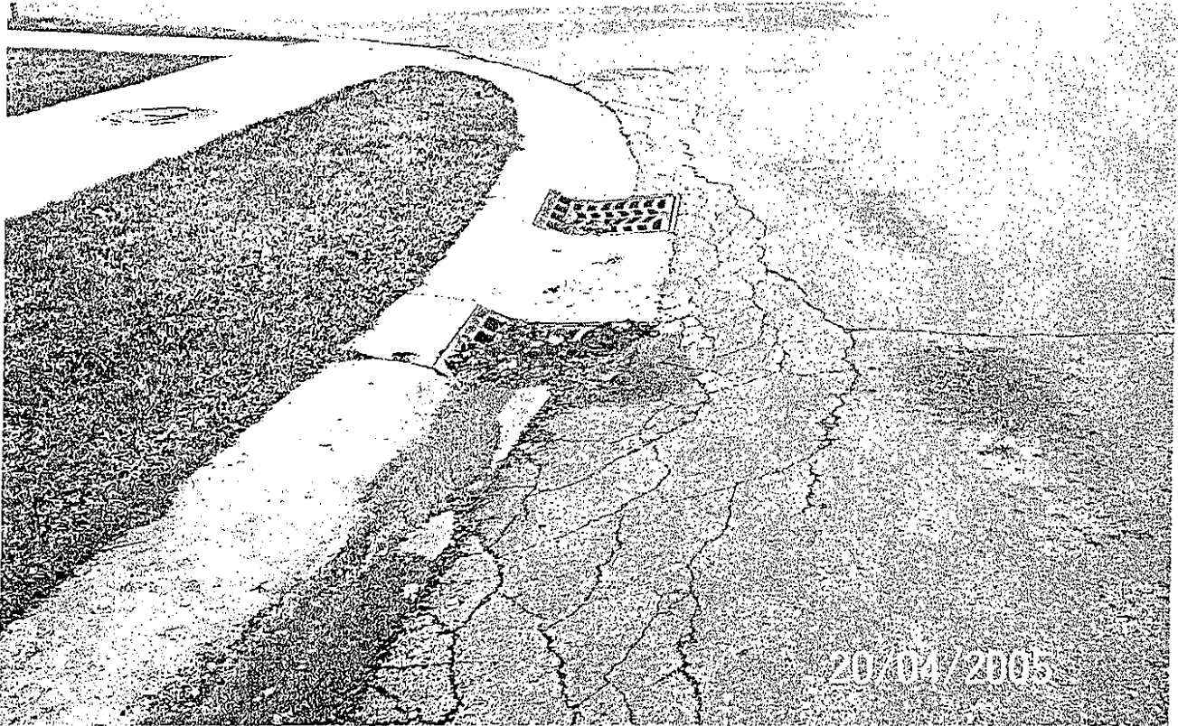
Ledgeview at Hearthstone Pot-hole has formed in front of catch basin and edge cracking. The cracking continues into cul-de-sac on both sides of roadway.
