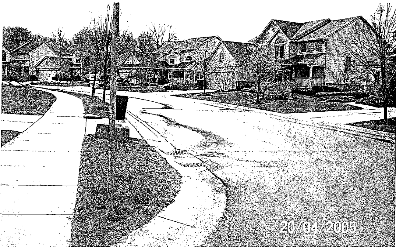
Sandstone east of Hearthstone Heaved pavement is causing storm water to pond on road surface. Surface cracks have formed in location where pavement has heaved and at the catch basins.
