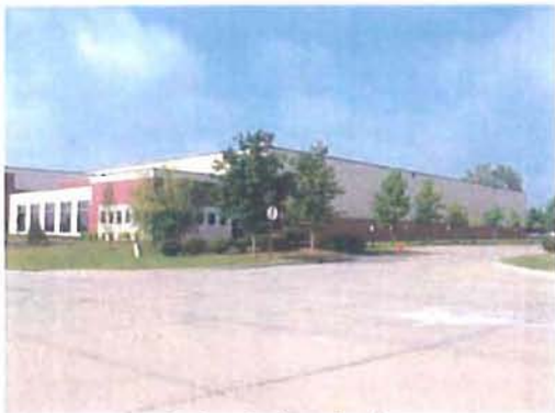
Exterior - Southwest Exterior
