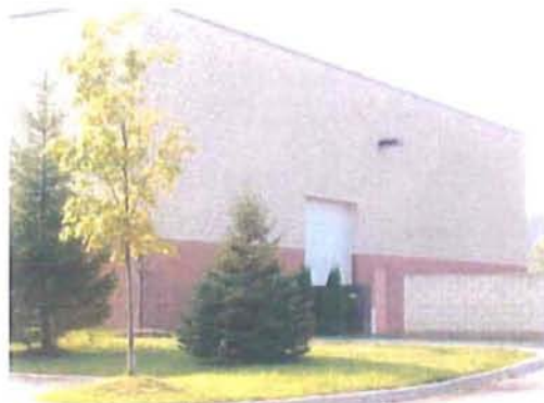
Exterior - Rear of Building
