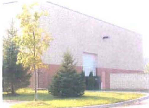
Exterior - Rear of Building
