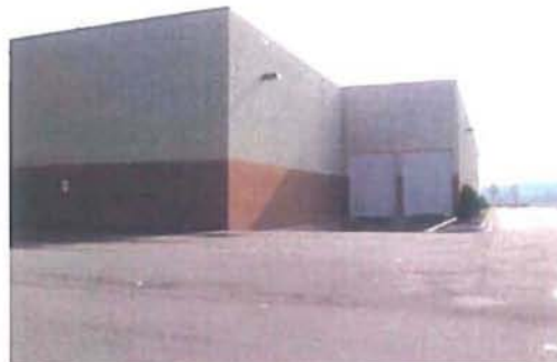
Interior - Loading Dock
