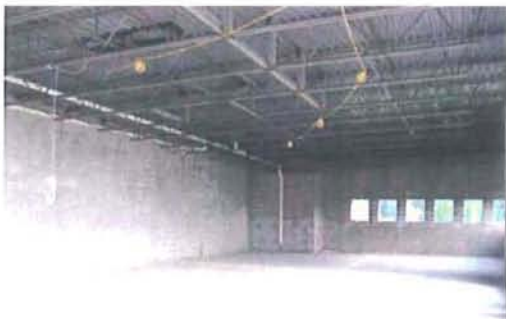
Interior - Unfinished Office Space
