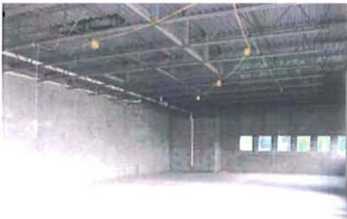
Interior - Unfinished Office Space
