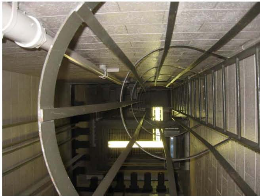
Photograph No. 2 Hose drying tower interior.
