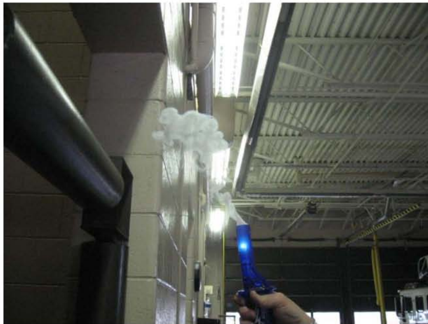
Photograph No. 4 Smoke from puffer being drawn into hose drying tower.
