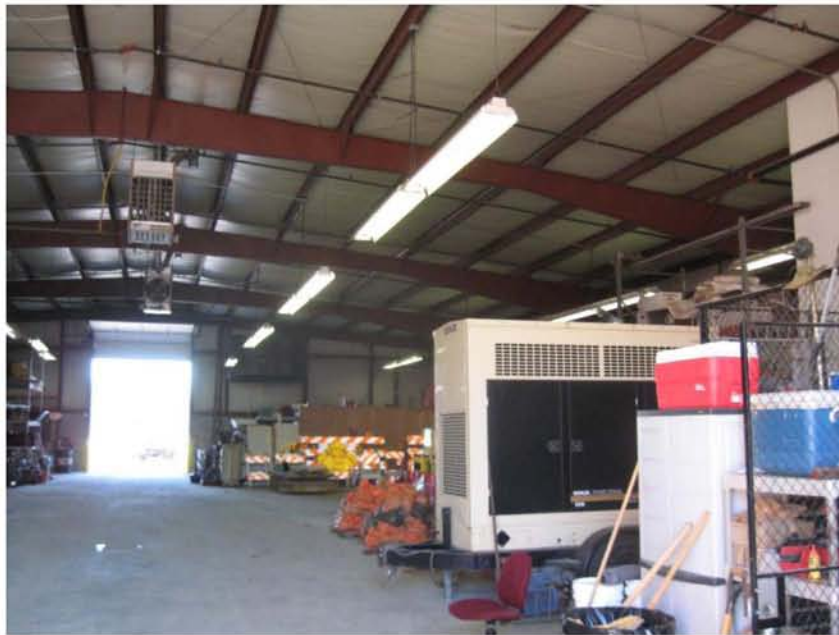
Photograph No. 12 Interior of DPS storage facility. Automatic door closers and occupying sensors needed for lighting.
