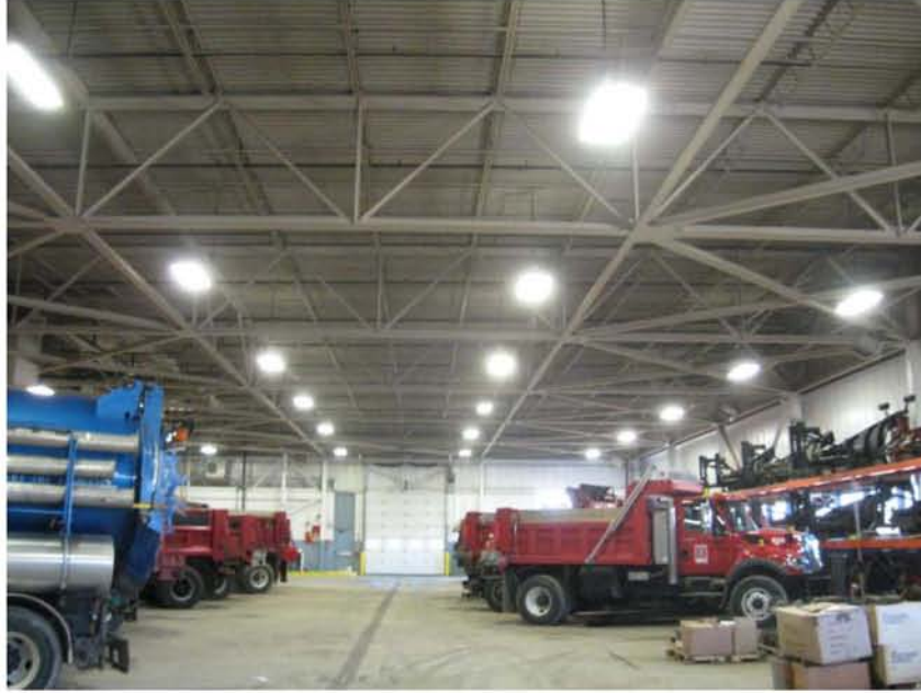
Photograph No. 1 Truck bay for field service complex.
