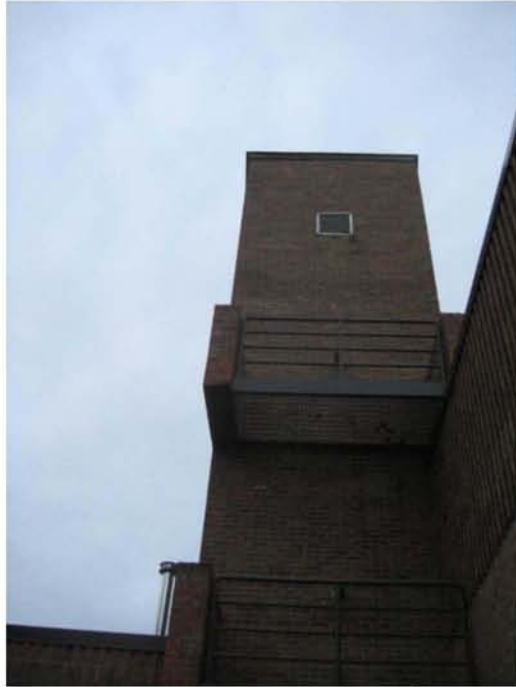
Photograph No. 1 Hose drying tower exterior.
