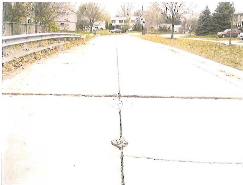
Typical condition of deck surface – Northbound lanes shown
