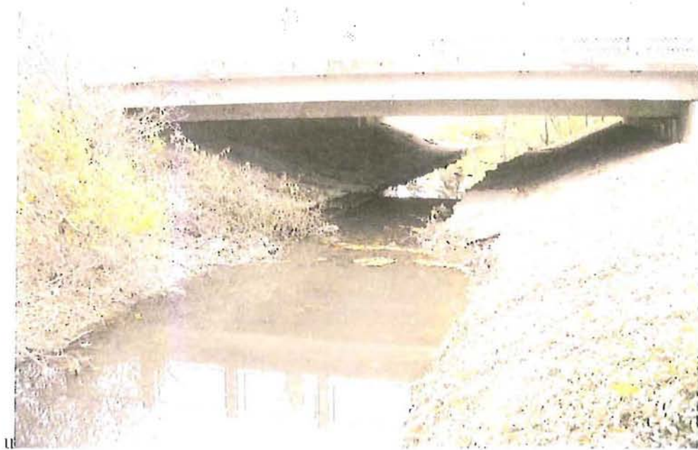
Cranbrooke Drive over Courter Ditch – East Fascia shown
