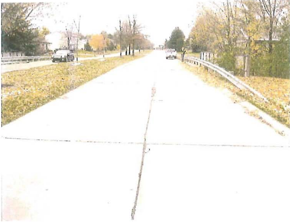
Typical Approach Pavement Condition
