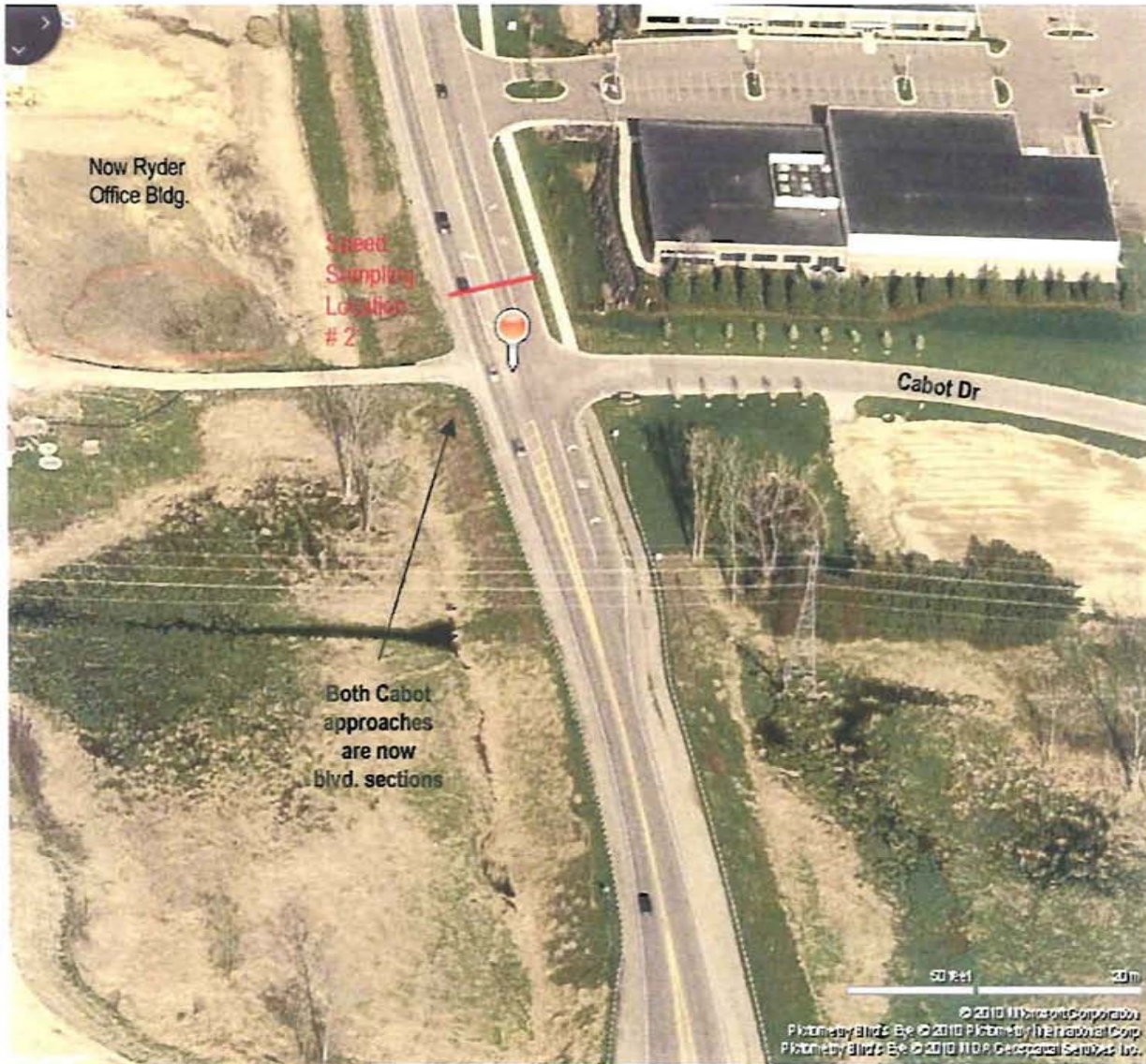
Figure 6. 13 Mile Road at Cabot Drive
