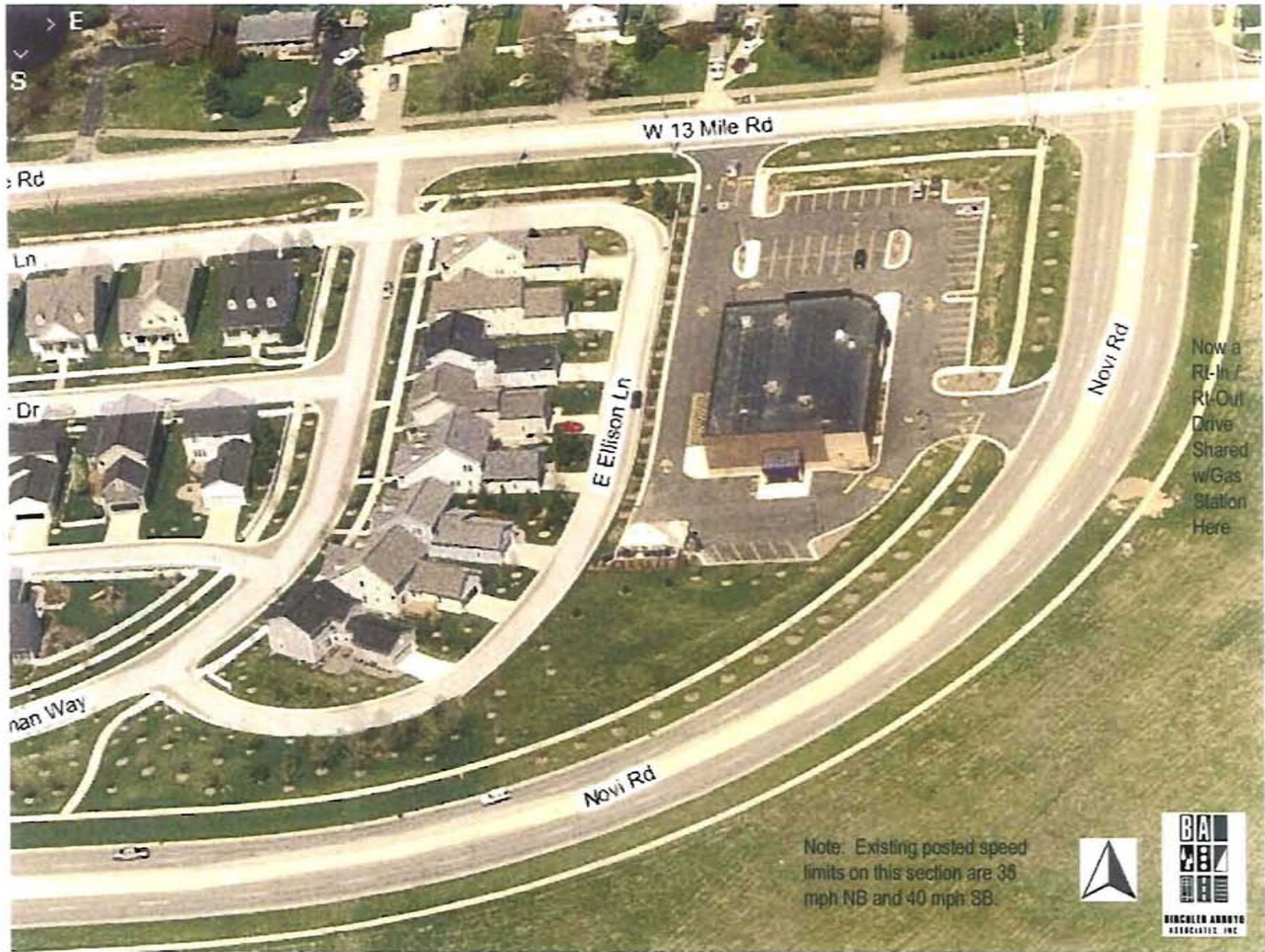
Figure 10. Novi Road, From 13 Mile South Through First Curve
