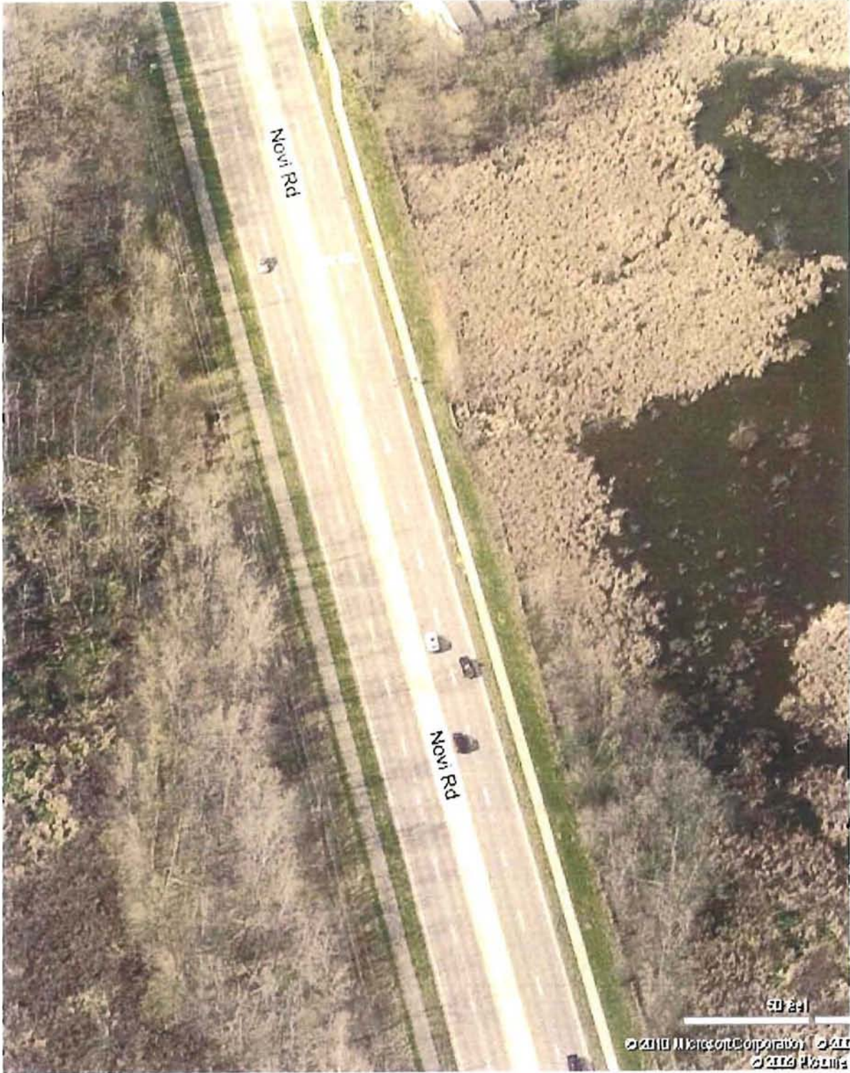
Figure 6. Novi Road, Fourth Section South of 14 Mile
