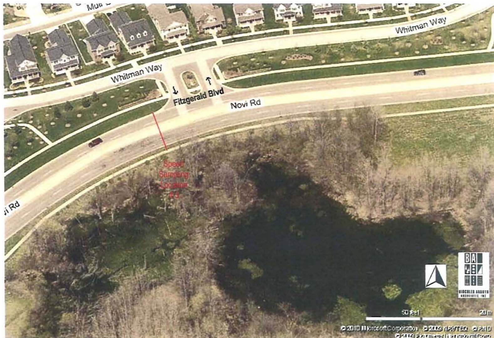
Figure 11. Novi Road, Second Section (and Curve) South of 13 Mile
