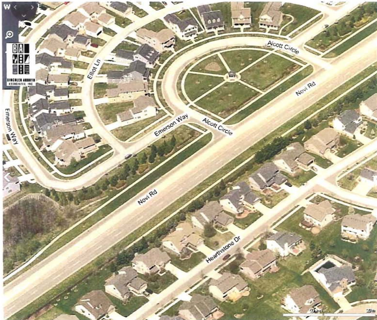
Figure 13. Novi Road, Fourth Section South of 13 Mile
