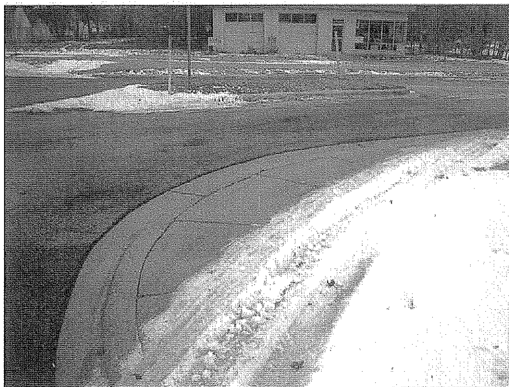
Figure 8. Off-Tracking Apron at Entrance to South Lake Drive
