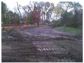
The rough grading of the secondary spillway is under way. The construction includes a buried concrete control structure at the edge of the lake to control the lake level at the overflow spillway, set to pass high frequency 2-year storms. This is to allow smaller storm events to bypass the primary dam structure and increase the capacity of the dam to meet DEQ requirements for a 100-year storm.
