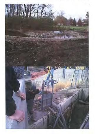
Rip rap was installed along the stream banks of the river channel to better prevent stream bank erosion.
