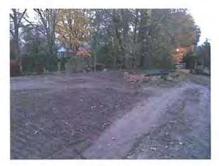
The earthen embankment for the dam was re-graded (east side shown here) to improve the safety of the dam to decrease the chance of overtopping the embankment and causing failure of the dam. A majority of the on-site subgrade clay soils were sufficient to construct the proposed berm to meet MDEQ specifications.
