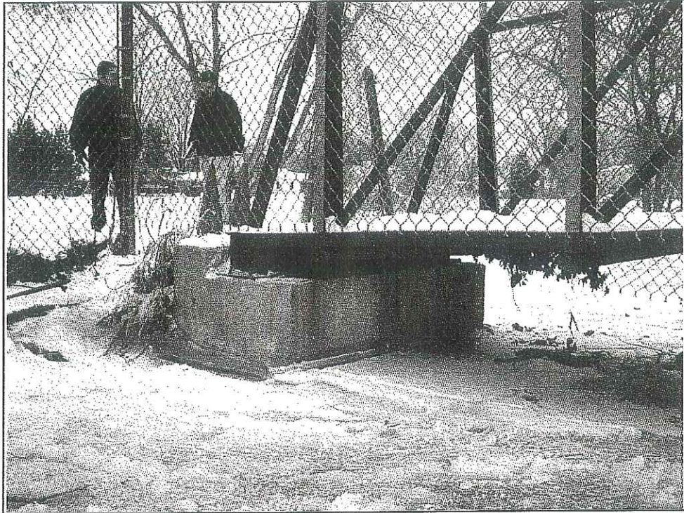
Picture 3 – North half of west elevation
