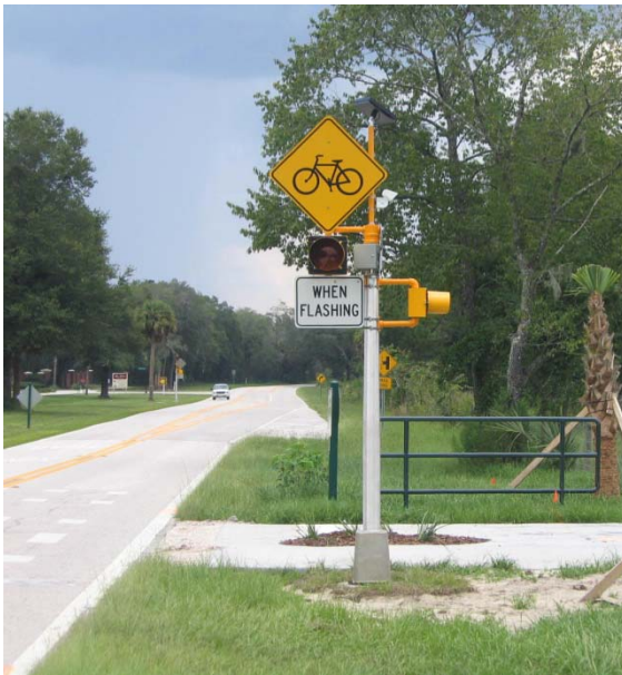
Fig. 5.7G. Active Crosswalk Warning Systems
