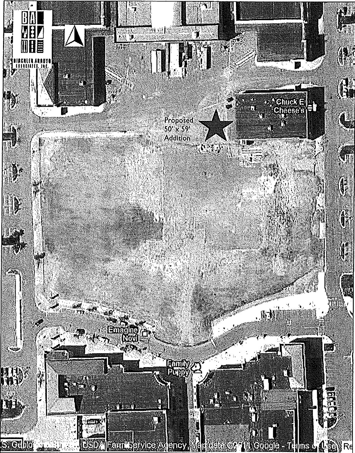
Location of Chuck E. Cheese #331 within North Portion of Twelve Mile Crossing at Fountain Walk
