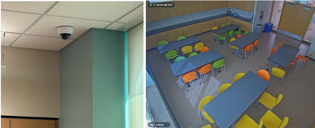
Security Camera #14 moved to YAR View from Camera #14
