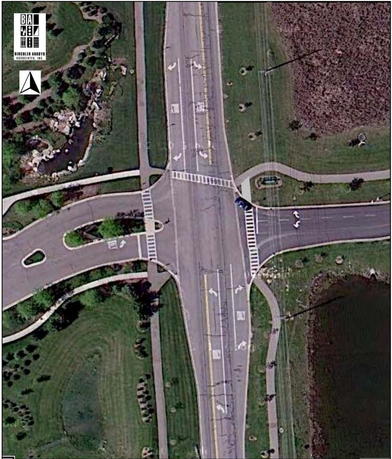
Figure 3. Intersection of Wixom Road, Glenwood Drive, and School Driveway
