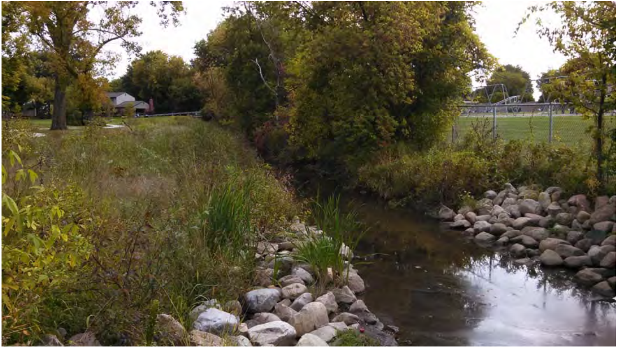
Streambank stabilization along Ingersol Creek
