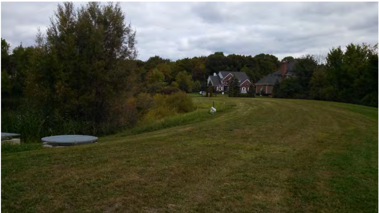
Improve maintenance access road for Thornton Creek Regional Detention Basin
