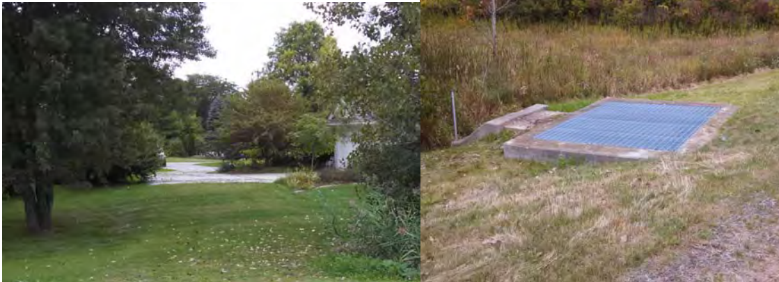
Improved outlet control and maintenance access at Leavenworth Regional Detention Basin.
