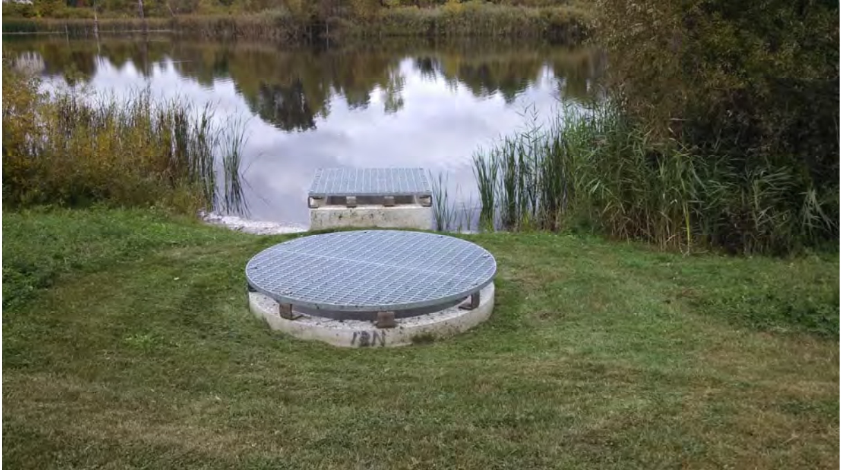
New outlet control and overflow for Thornton Creek Regional Detention Basin
