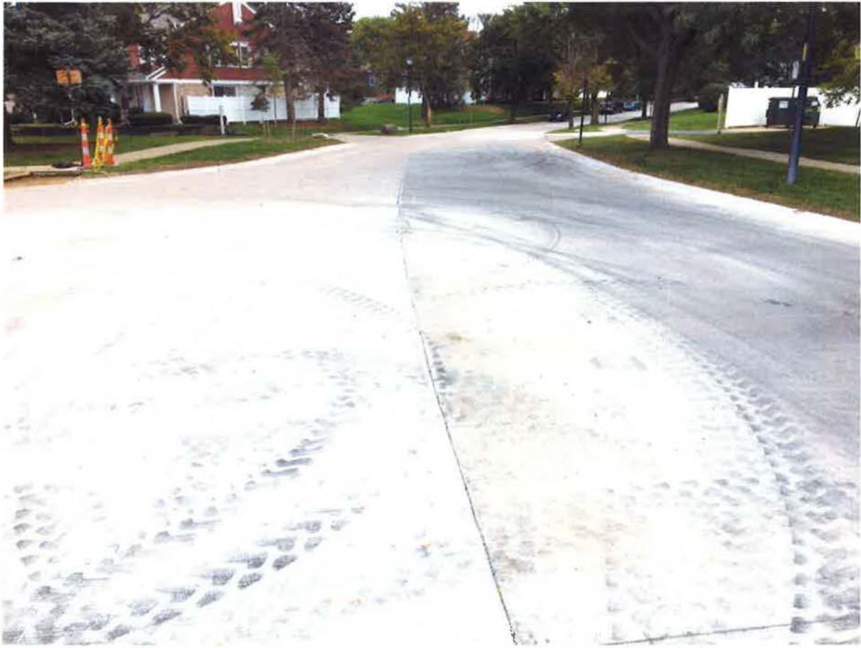
East Glen Haven – Looking east and south towards 8 Mile Road
