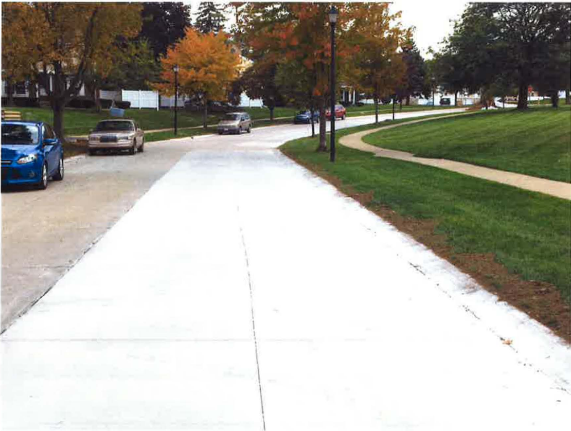
Glen Haven Circle East – Looking south towards East Glen Haven
