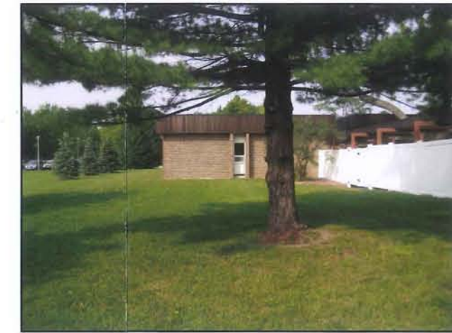
A-3 Courtyard Security Fence
