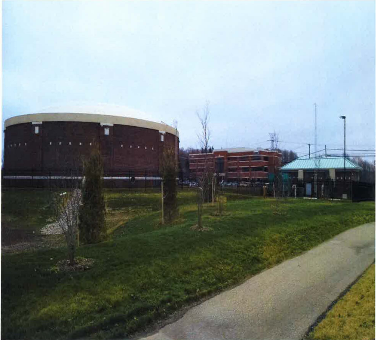
Overall Storage Reservoir and Station from West Park Drive
