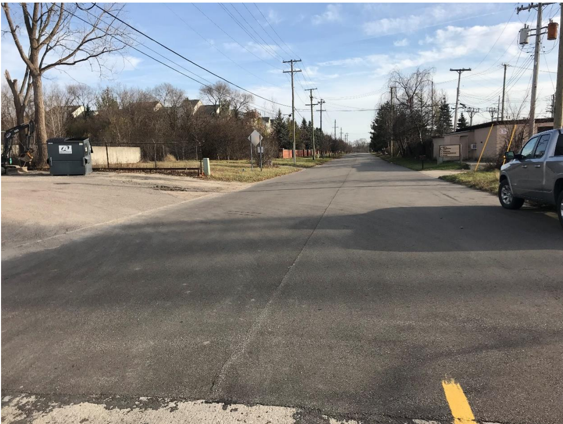
Trans-X Drive – Looking east from existing concrete portion of Trans-X/Novi Road
