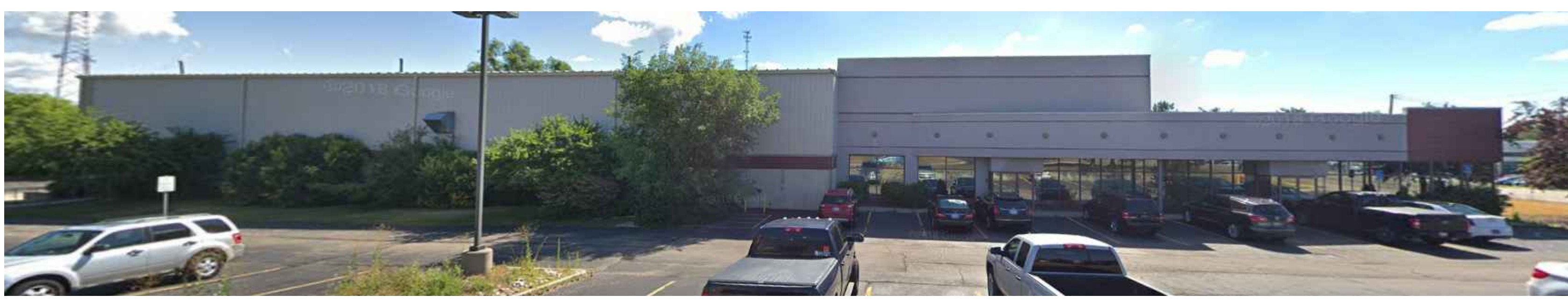
4 Existing Photo - West Elevation A2.01 SCALE: NTS REF:
