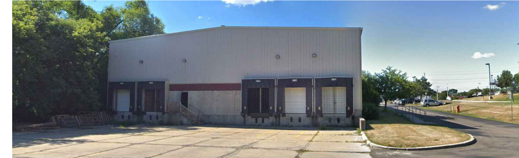
5 Existing Photo - North Elevation A2.01 SCALE: NTS REF:
