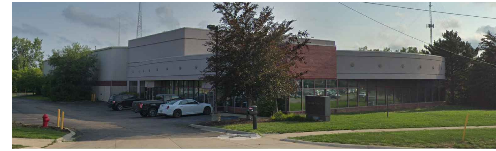
6 Existing Photo - S.W. Elevation A2.01 SCALE: NTS REF:
