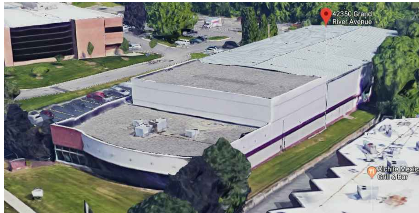
7 Existing Aerial - S.E. Corner A2.01 SCALE: NTS REF:
