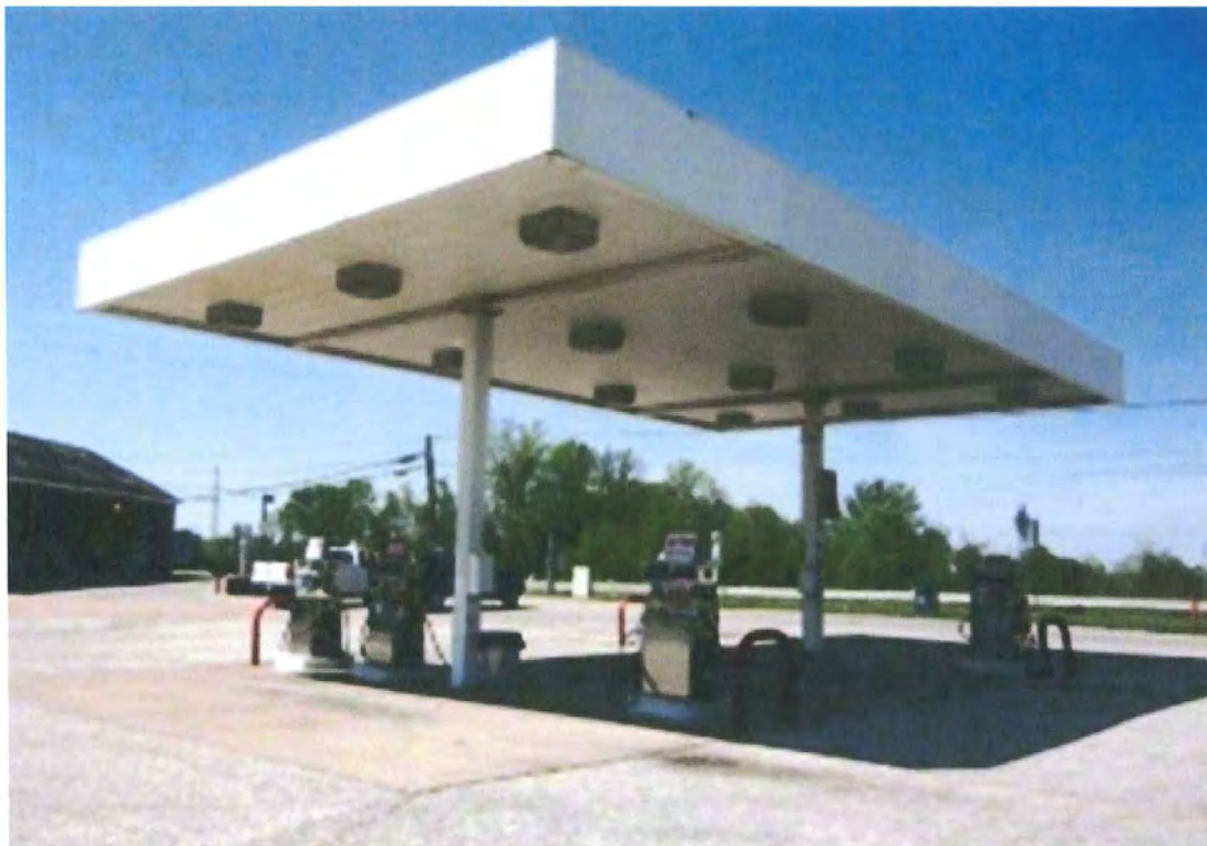
Sample photo of typical fuel island canopy during daylight
