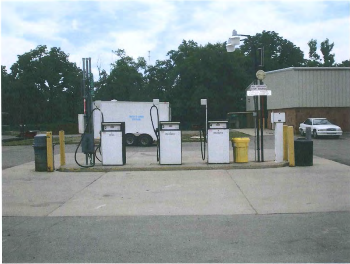
Existing Fuel Island
