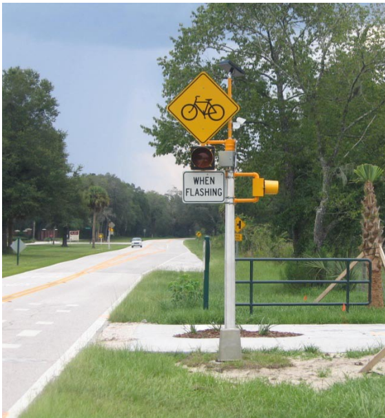
Fig. 5.7G. Active Crosswalk Warning Systems
