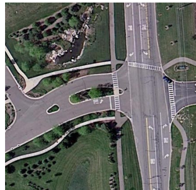
Raised Median at Glenwood Dr Entrance
