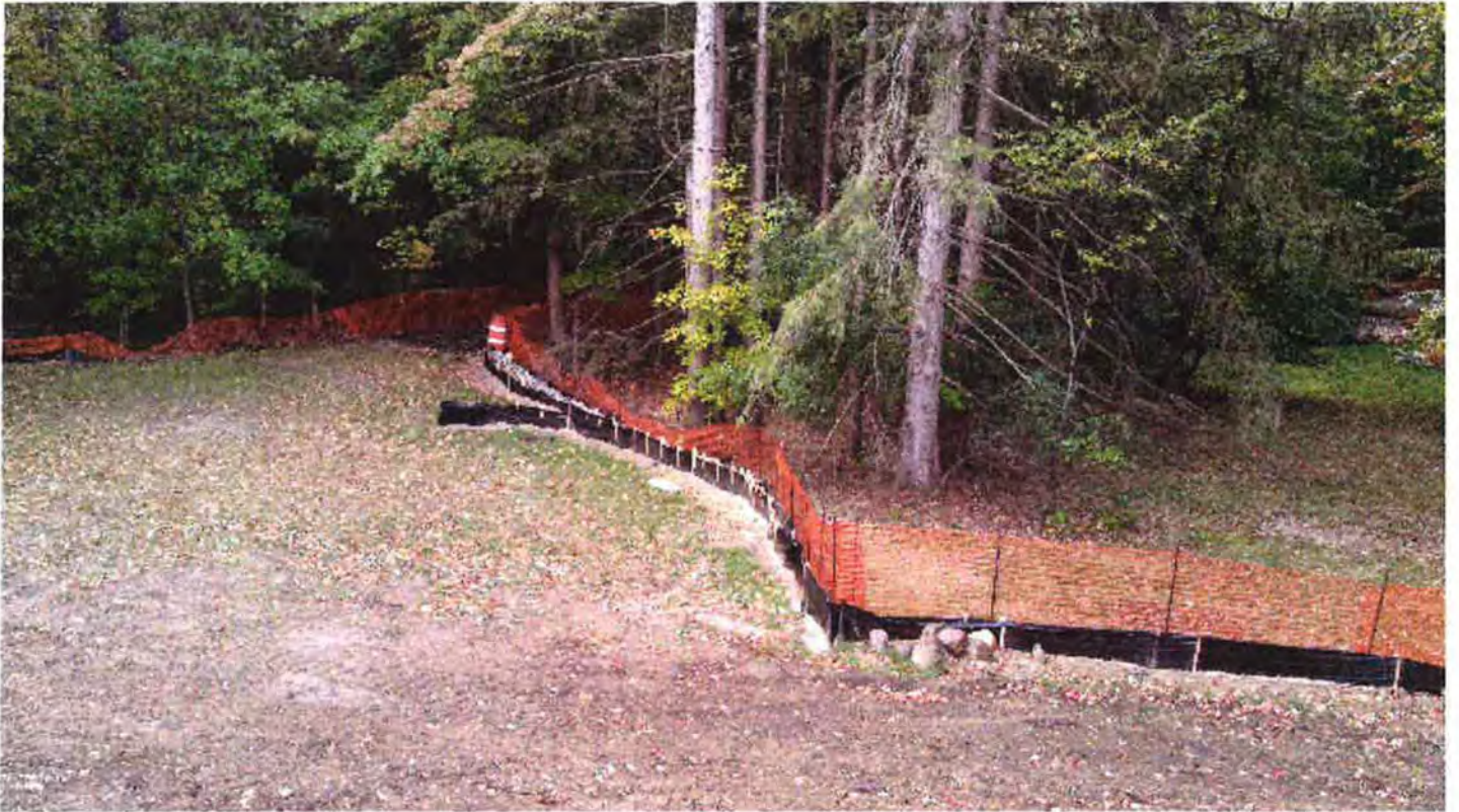
Silt fence beefed up behind lot 22 along the woods and wetland.
