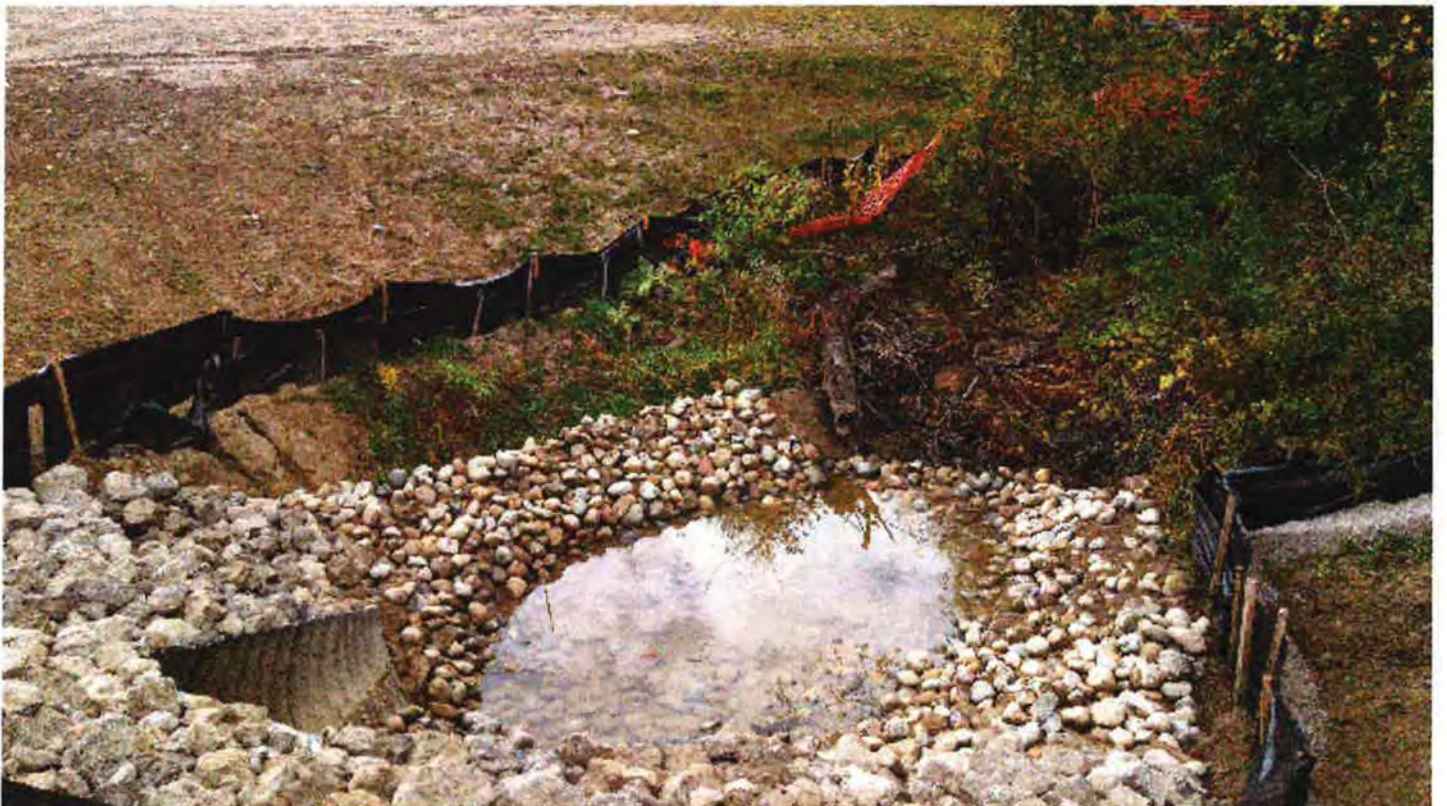
More creek stone was added at the Miller Creek culvert.
