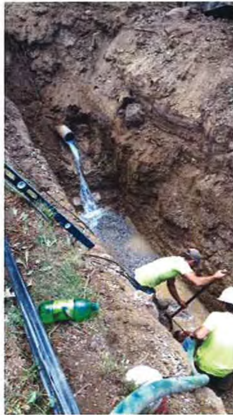
Cut off Existing 8" AC pipe
