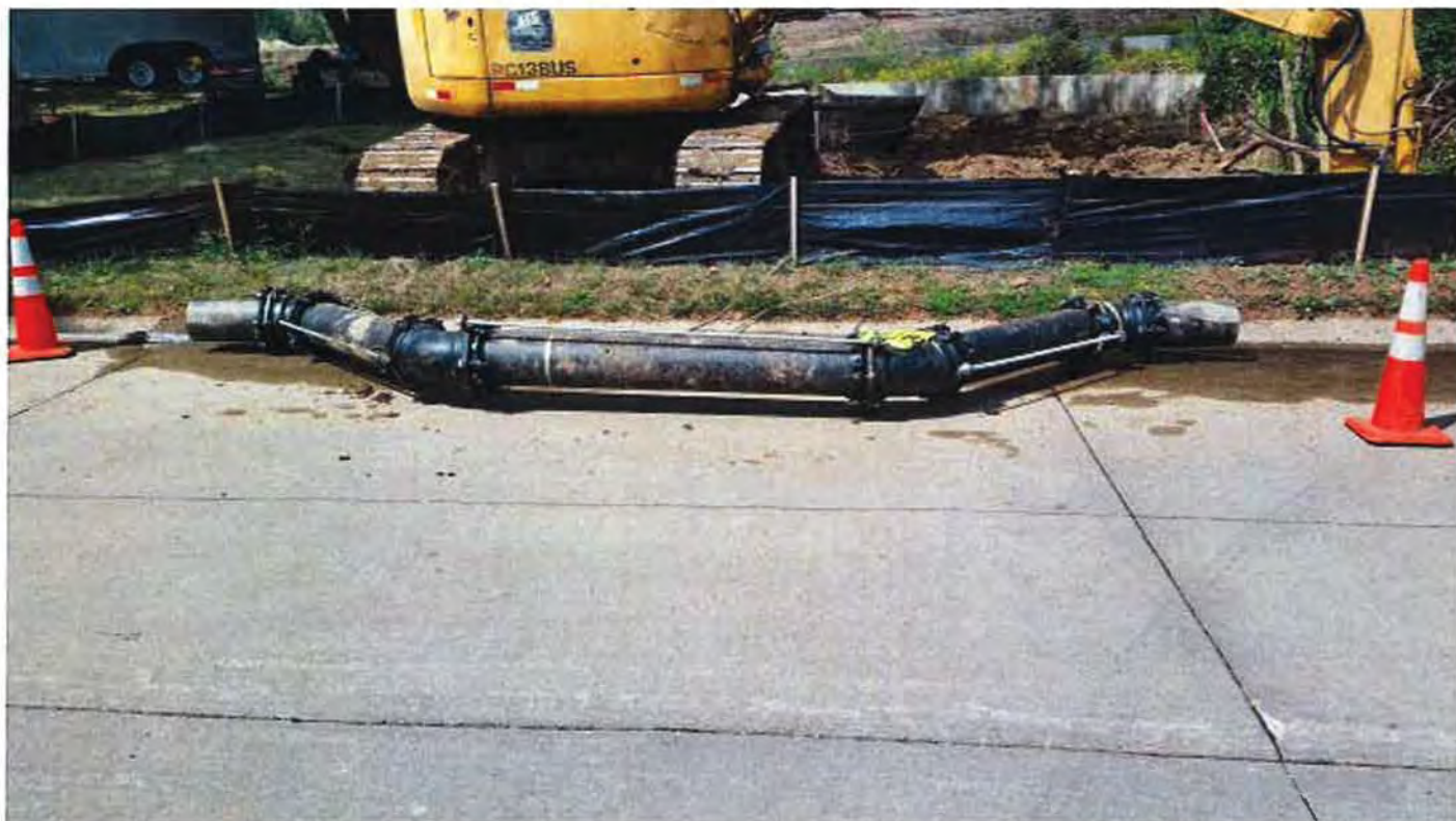
Assembled pipe, bends, restraints prior to attachment
