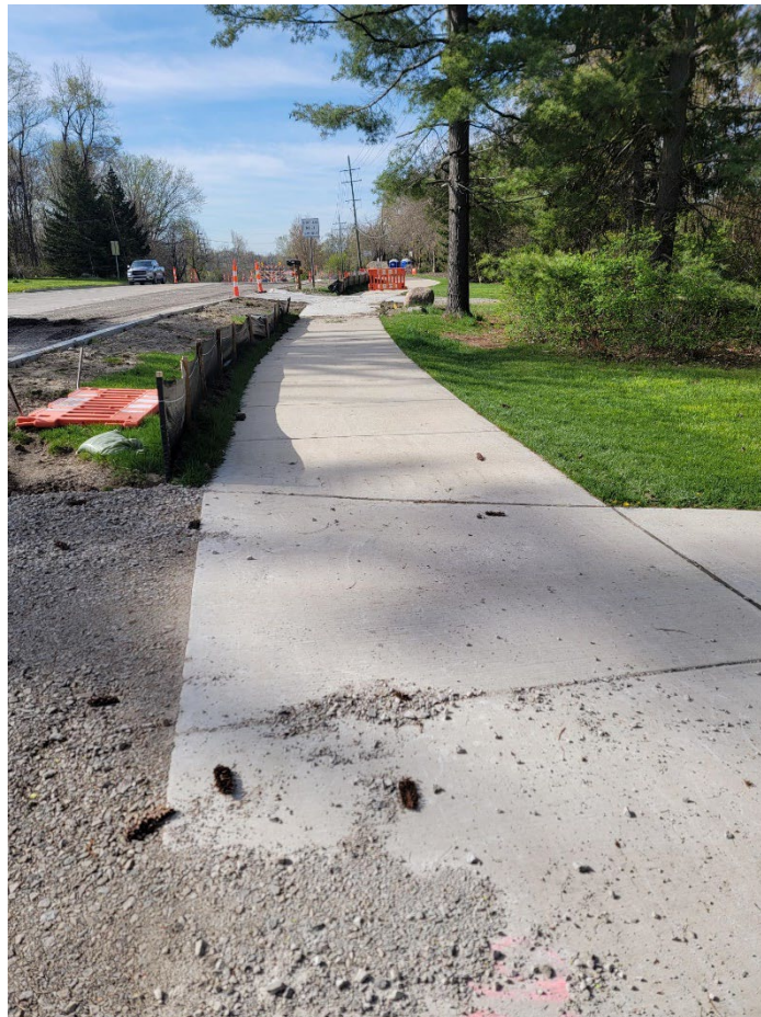
AFTER – Wixom Road Segment (Catholic Central to Island Lake Drive)
