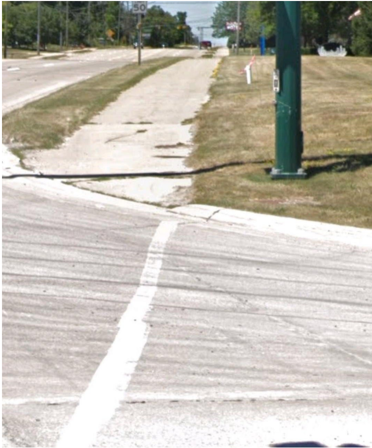
BEFORE – Grand River Avenue at Taft Road Intersection (north)
