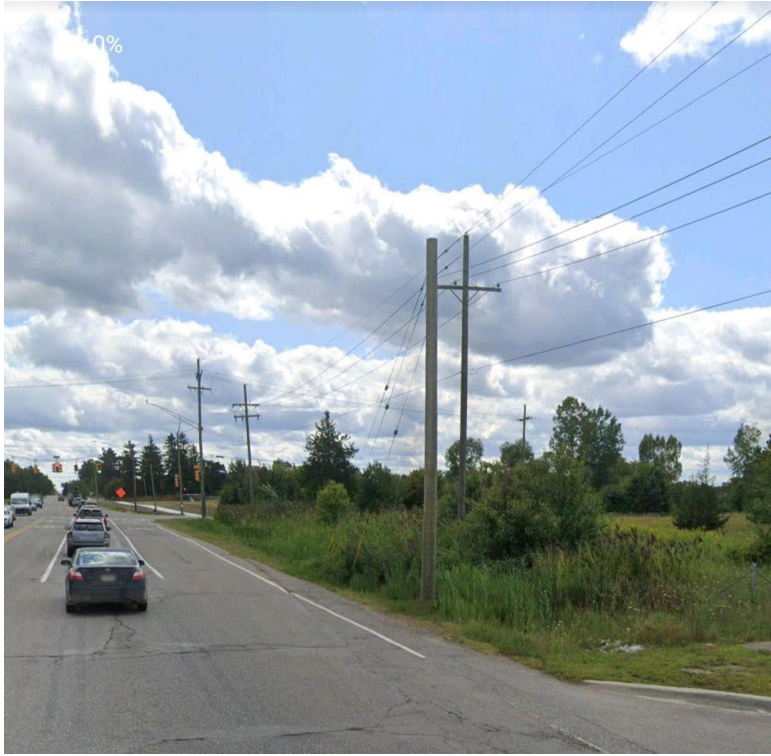
BEFORE - Beck Road Segment (11 Mile to Providence)
