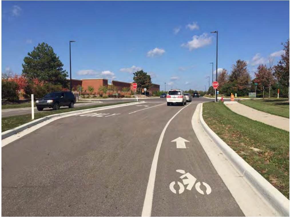
Town Center Drive Reconstruction with Bike Lanes
