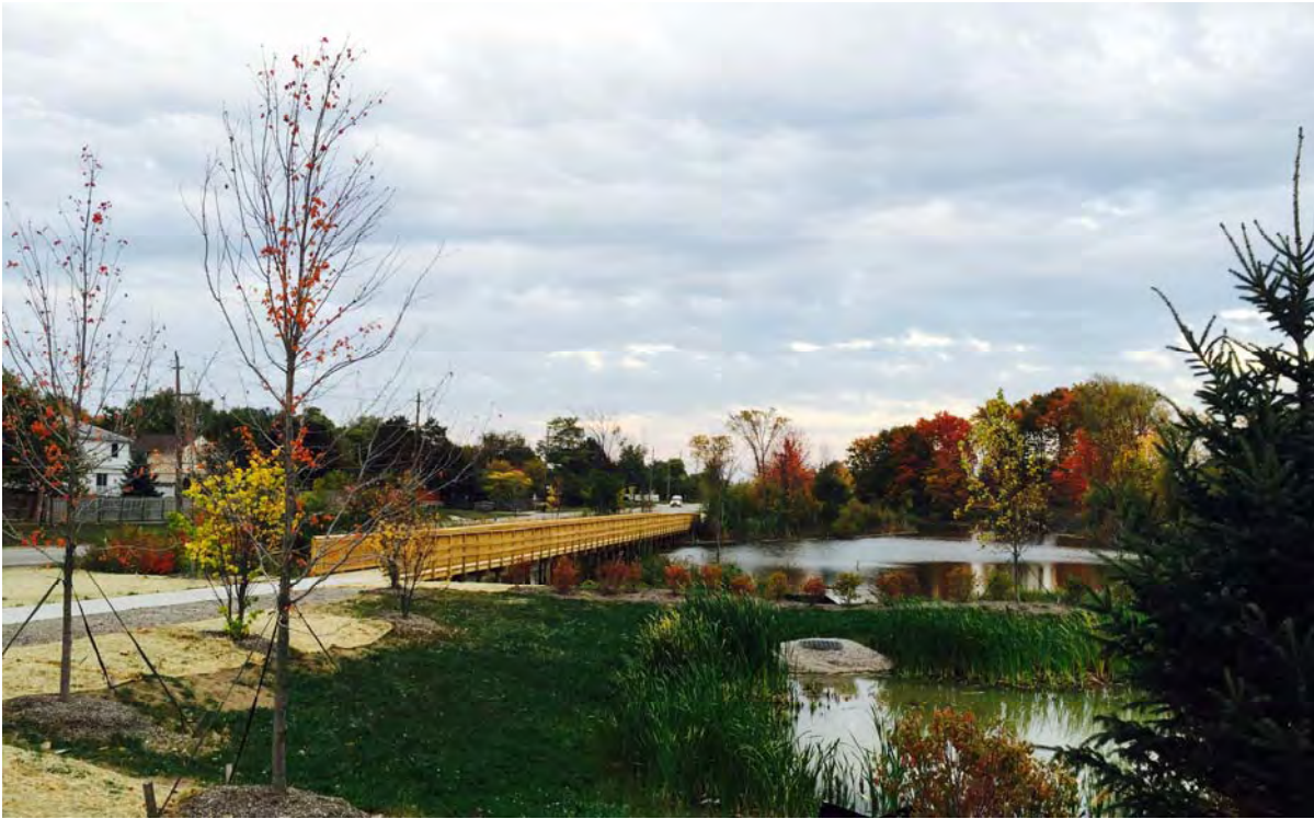
Completed Boardwalk along Ten Mile Road Protecting the Wetlands
