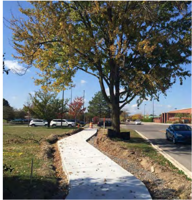
Sidewalk under construction in Town Center Area
