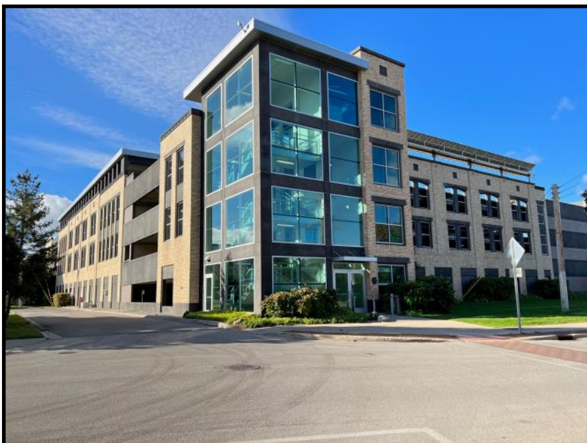
Figure E26: Parking structure in Traverse City
