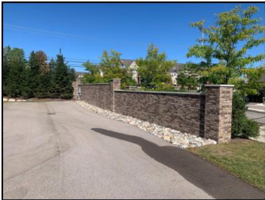
Figure E10: Huntley Manor Apartments in Novi has screening that separates Grand River, a major arterial, from residential units. Both decorative walls and landscaping in the form of trees were used to screen the homes from the street.
