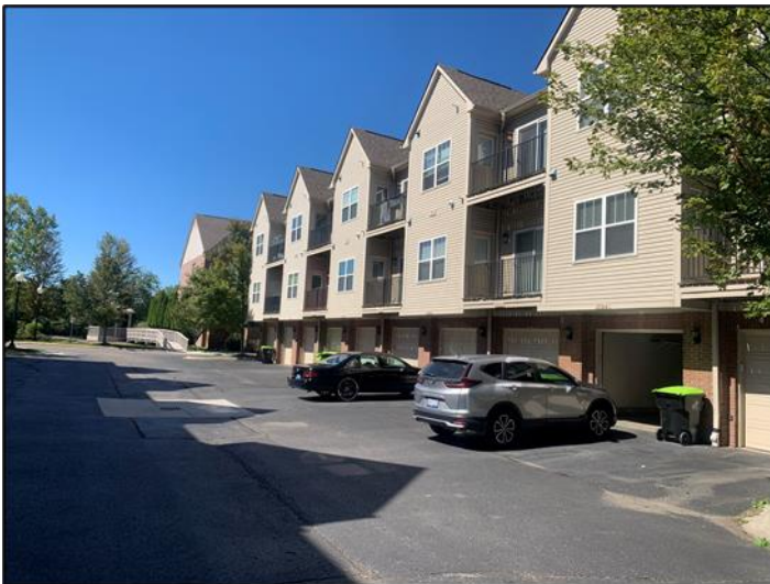
Figure D16: Gateway Townhomes in Novi have garage parking situated in back of the units
