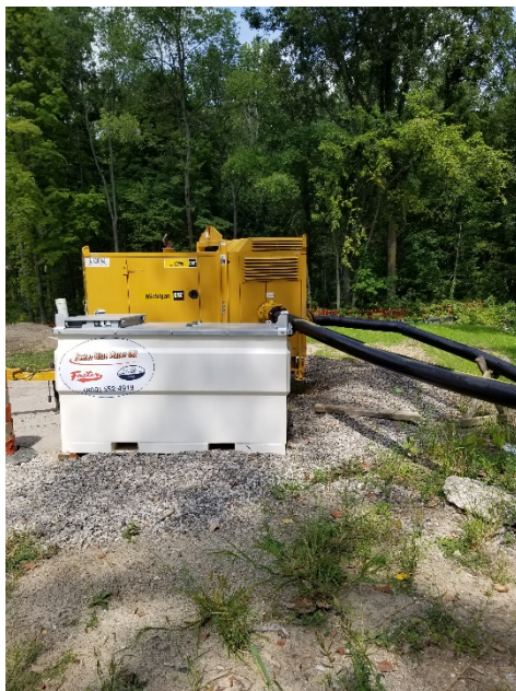
Pump used to direct water
