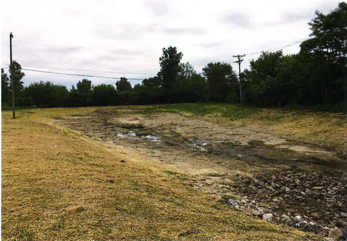
Heslip Basin – Post Construction – Looking north
