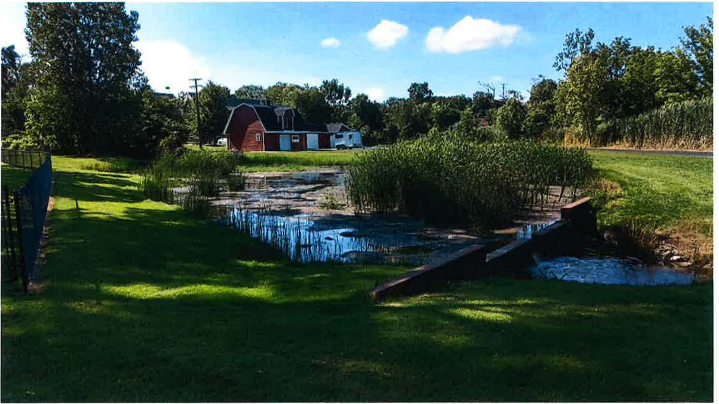
Bassett Drain (McSweeney Pond) – Pre-Construction Condition
