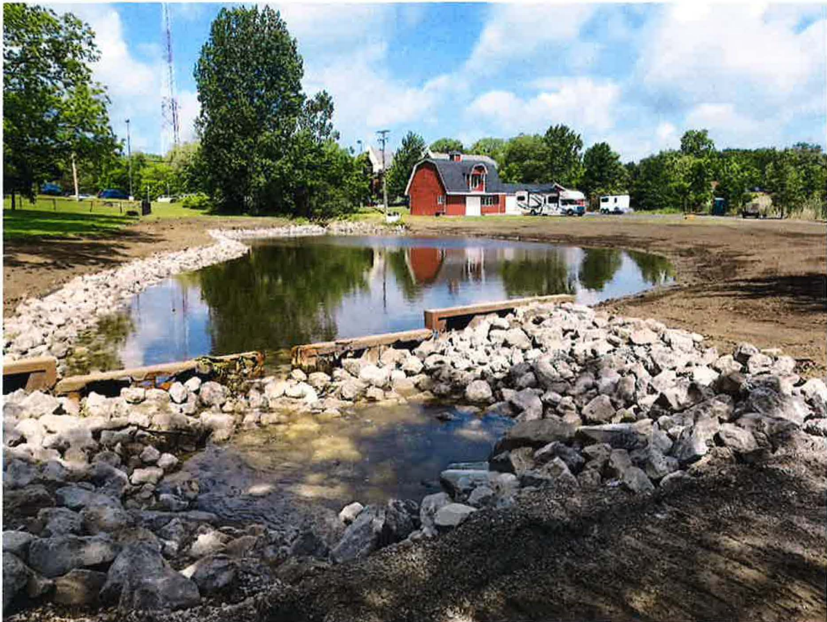
Bassett Drain (McSweeney Pond) – Post-Construction Condition
