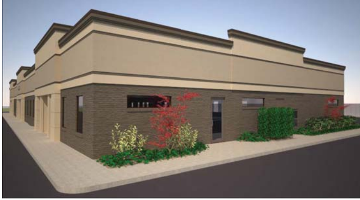
39555 - North / West View
