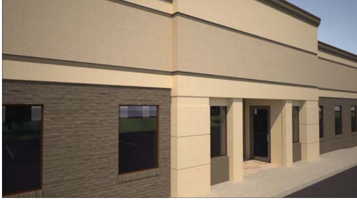
39555 - Typical Point of Entry
