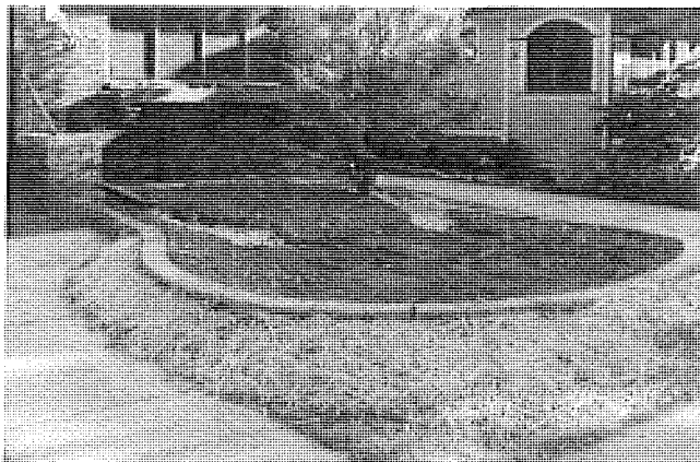
Use of Bioretention within a Residential Development
