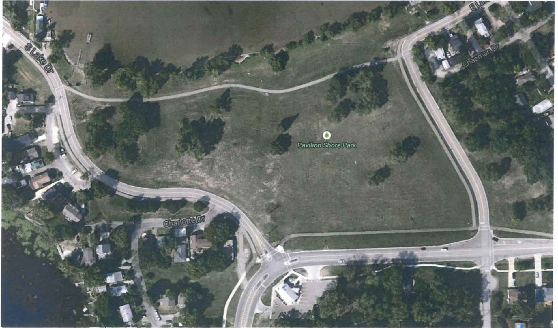
Previous Condition Pavilion Shore Park
