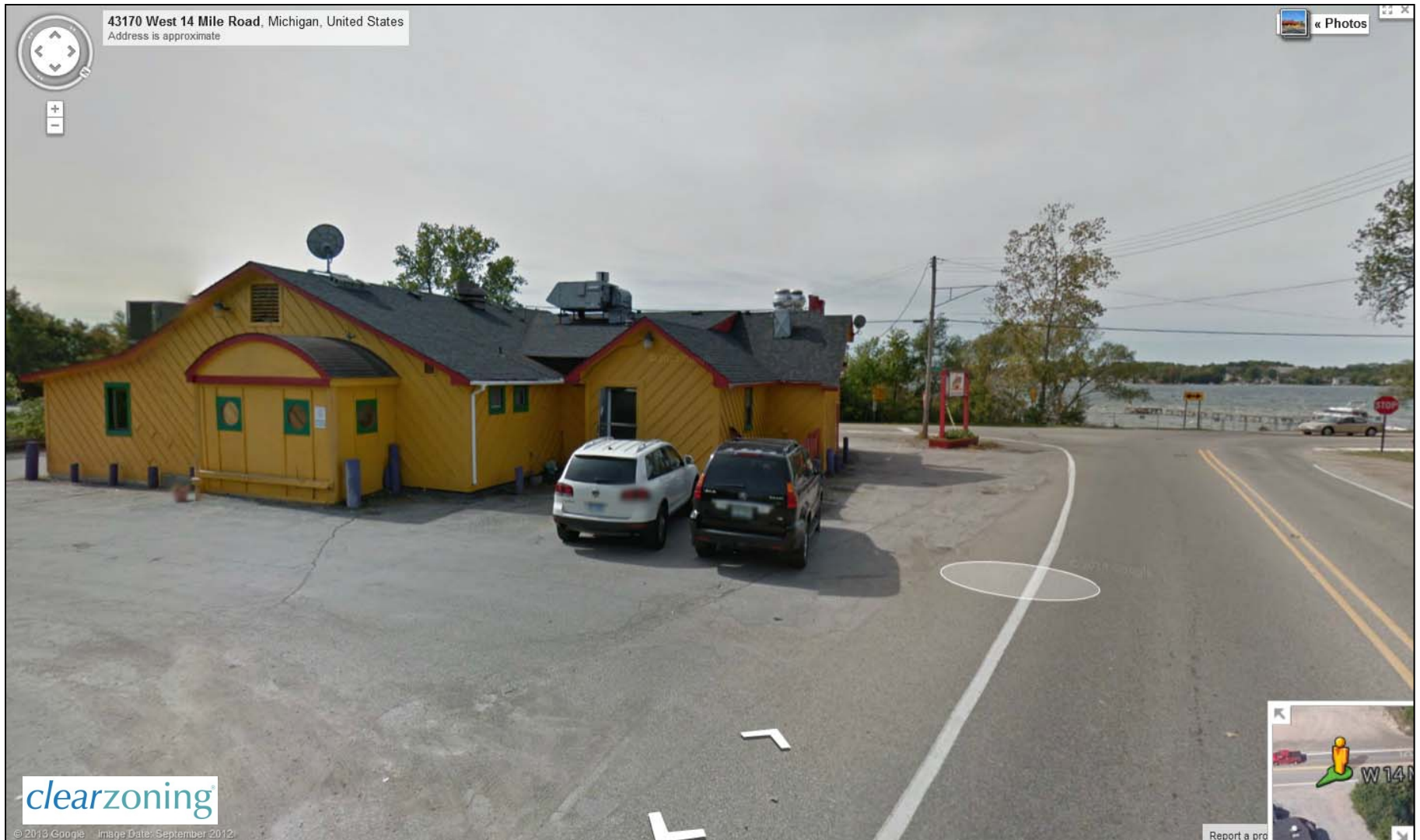
View of Existing Site from WB 14 Mile Road
