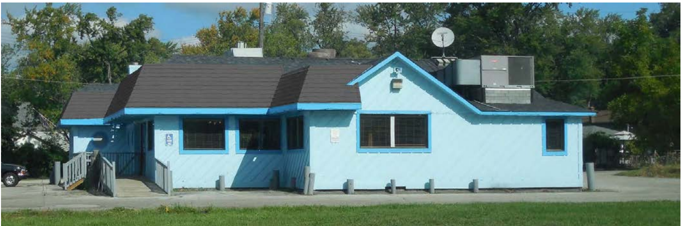
After as recommended with painting of asphalt shingles
