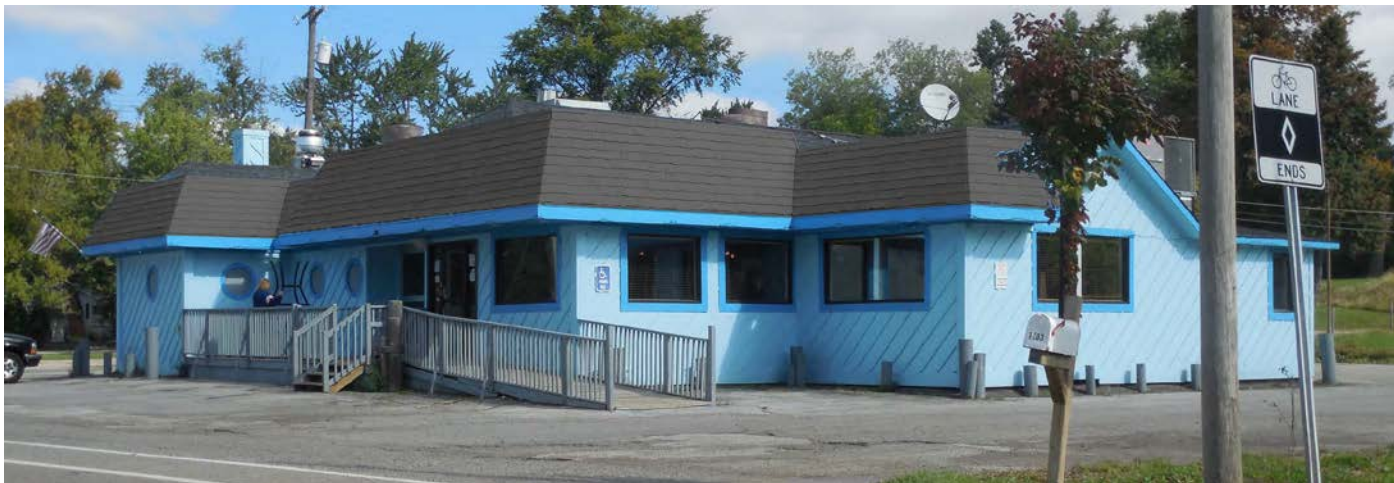
After as recommended with painting of asphalt shingles
