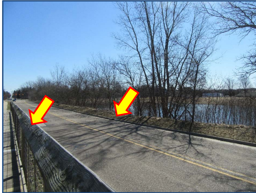
Photo 3. View east along W. Eleven Mile Road in area of existing 18" storm sewer and end section located at northwest side of the pond/wetland. Storm sewer curb inlets are indicated (ECT, March 22, 2017).
