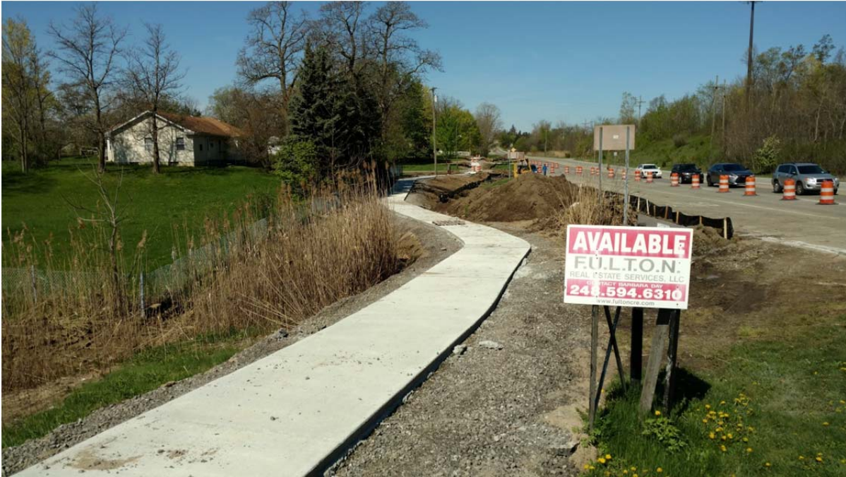
Looking west along sidewalk along south side of Fourteen Mile Road.
