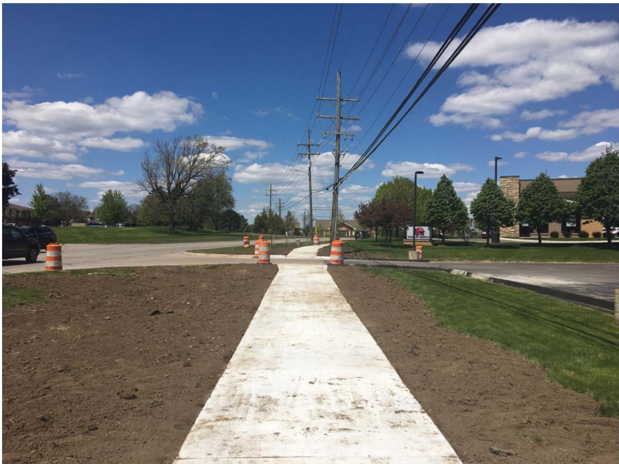
Looking north along new sidewalk along east side of Beck Road.
