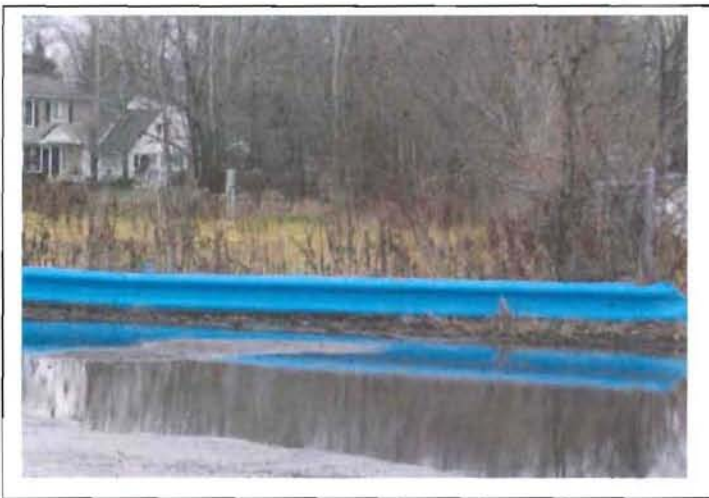
GUARD RAIL (12/4/12) (9/24/13 – GUARDRAIL HAS BEEN ELIMINATED)
