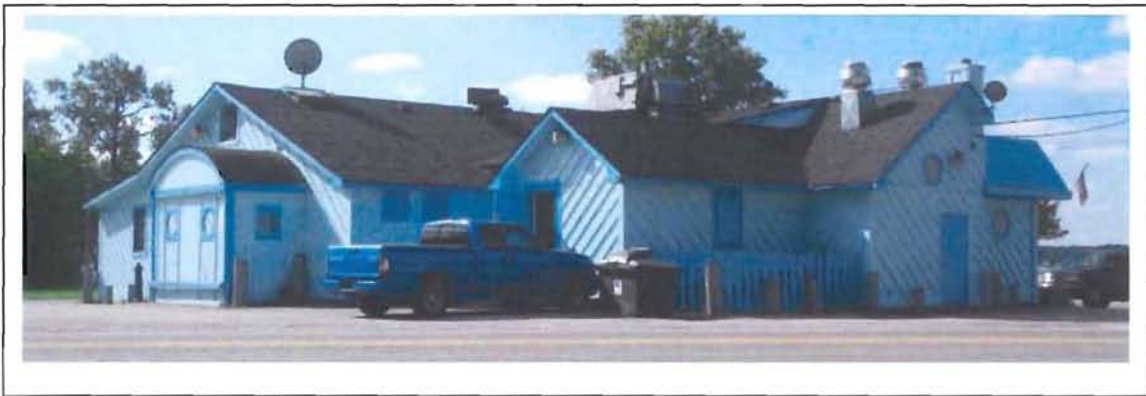
EAST & NORTH FACADES (9/24/13)
