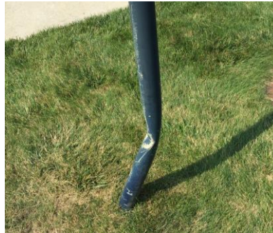
Figure 9: Damage to Sign Post at Island Lake Drive and Seaglen Drive
