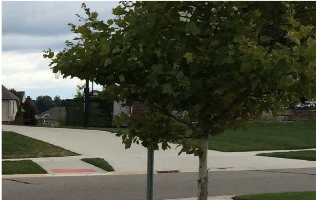
Figure 11: Existing Yield Sign Concealed by Tree at Calvert Isle Drive and Amesburg Drive
