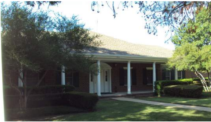
Celestial Road Pump Station
