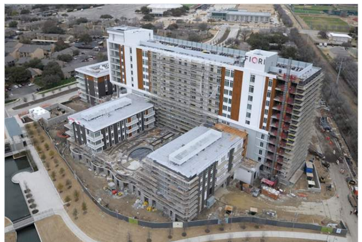
The Fiori at Vitruvian Park, currently under construction.
