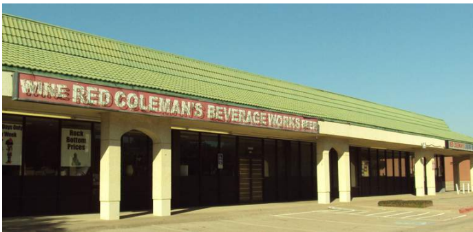
Closed liquor stores on Inwood Road.
