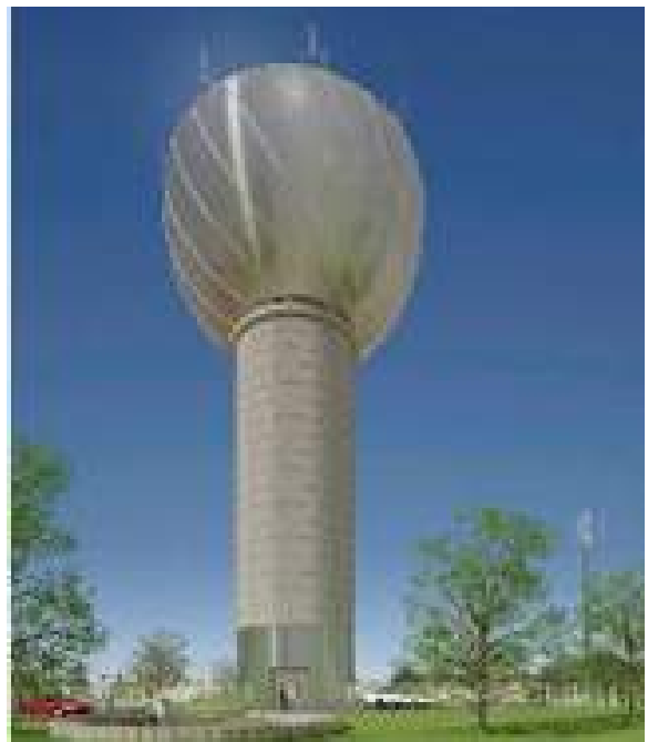
The new Elevated Tank at Surveyor Blvd.
