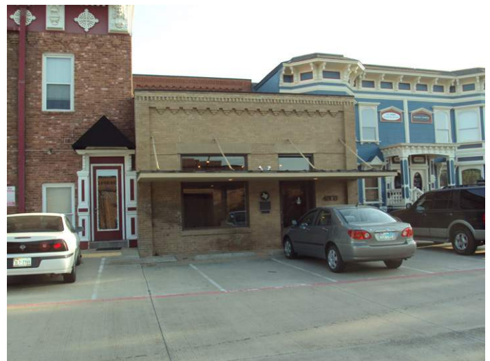
The Addison State Bank building today.
