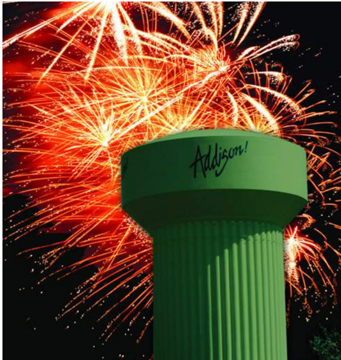
Addison Circle Elevated Tank
