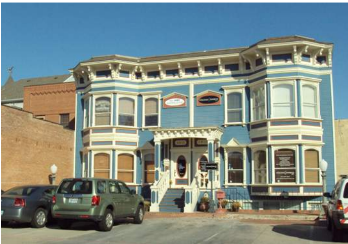
Victorian-style building in Old Addison.
