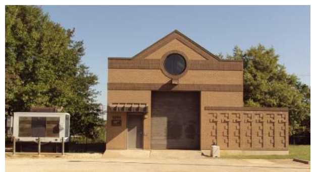
Kellway Circle Sanitary Sewer Lift Station
