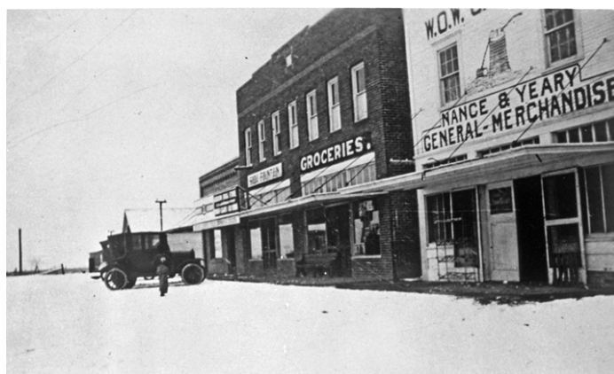
The original "Town" of Addison. One building, the original Addison Bank, still stands along Broadway, formerly the only commercial area in the community.
