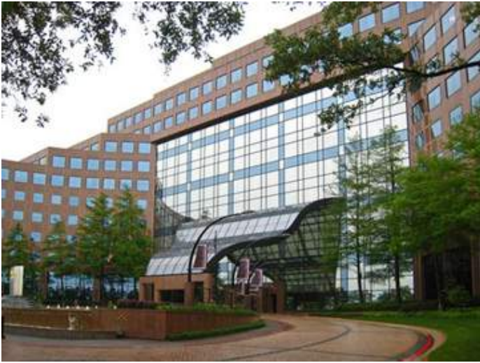
The Mary Kay Corporation headquarters, located on the Dallas Parkway.
