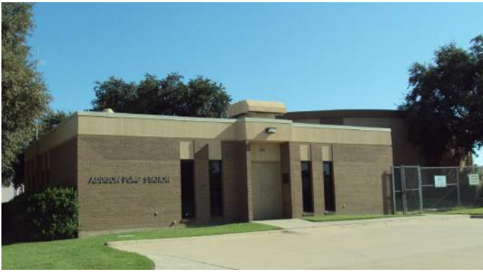
Surveyor Above-Ground pump station at Surveyor and Arapaho
