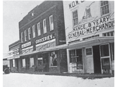
Addison State Bank (far building).
