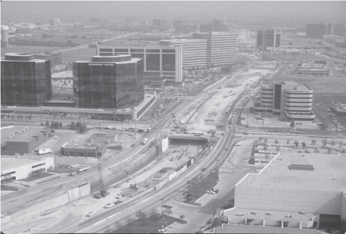
Construction of the Dallas North Tollway through Addison. The Town paid to construct the Tollway underground so that it would not cut the community in half.
