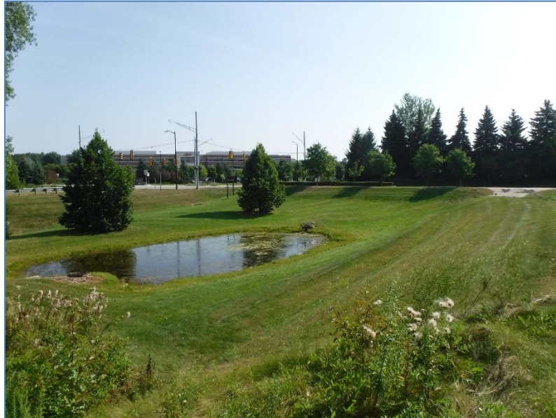
Photo 5. Looking north at the existing detention basin. ECT suggests that the applicant consider providing native vegetation within the 25-foot setback from this stormwater basin, as opposed to sod or common grass seed (ECT, August 12, 2019).
