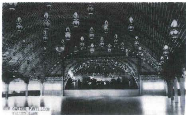
Figure 3: Interior of former casino/dance hall
