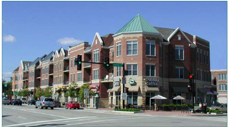
The Lofts at Village Center in Mt. Prospect, IL is a small-scale mixed-use building. It includes 34 loft-style condominiums ranging in size from 825 to over 2,075 square feet. The top floor apartments include vaulted and cathedral ceilings. The first floor includes over 23,000 square feet of retail. Resident parking is provide in the basement, and is accessed via a shared below-grade garage which is shared with the adjacent building. This project was designed by architect Matthew Haylock of Gurnee, IL.
