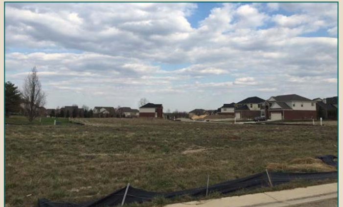
View from the subject property looking towards the single family homes to the south. Build out of the development has recommenced following the Great Recession.
