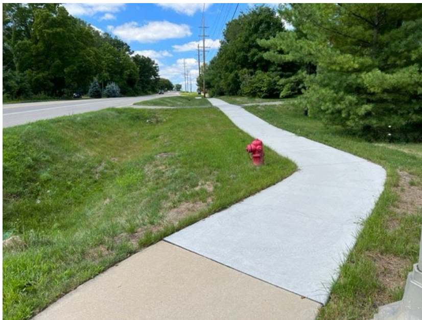
Segment 159 and 49: Two short segments built by the City west of Wixom completes connectivity on the north side of 10 Mile from Napier to Haggerty
