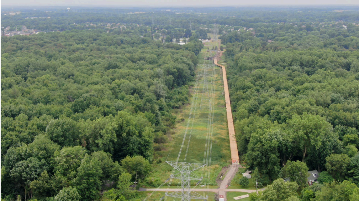
Longest Boardwalk in Novi, approximately 1,975 feet long (nearly 0.4 mile) is part of the ITC Trail
