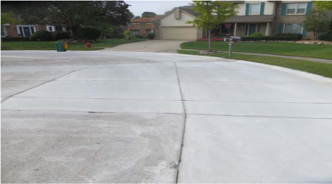
Simmons Drive looking North after repairs
