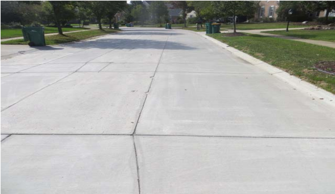
Fairway Hills Drive looking North after repairs
