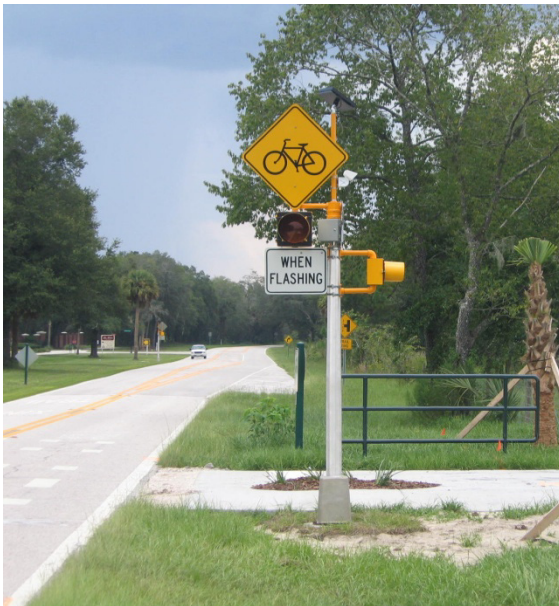
Fig. 5.7G. Active Crosswalk Warning Systems
