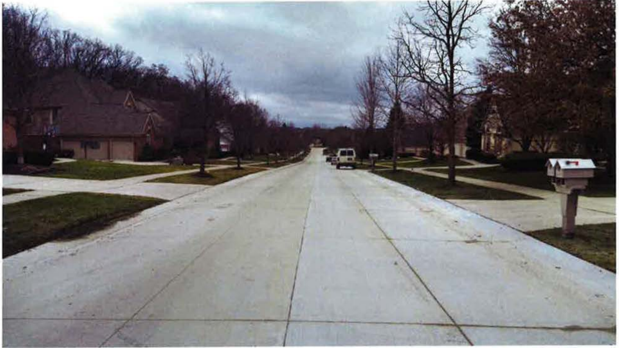
Chase Drive, looking southwest towards Trent Court.
