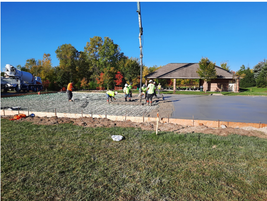
Pickleball Courts – Formed and poured with fresh concrete at south end.
