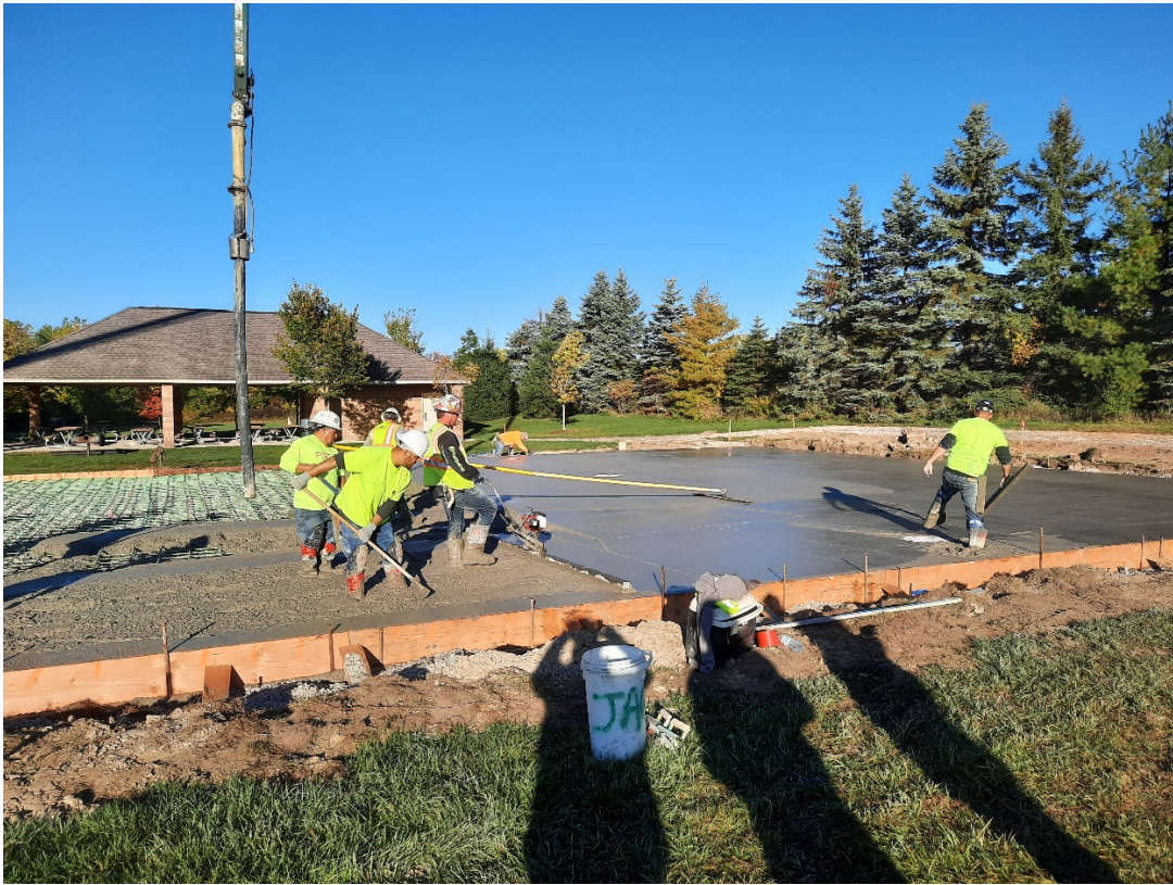
Pickleball Courts – Formed and poured with fresh concrete at north end.
