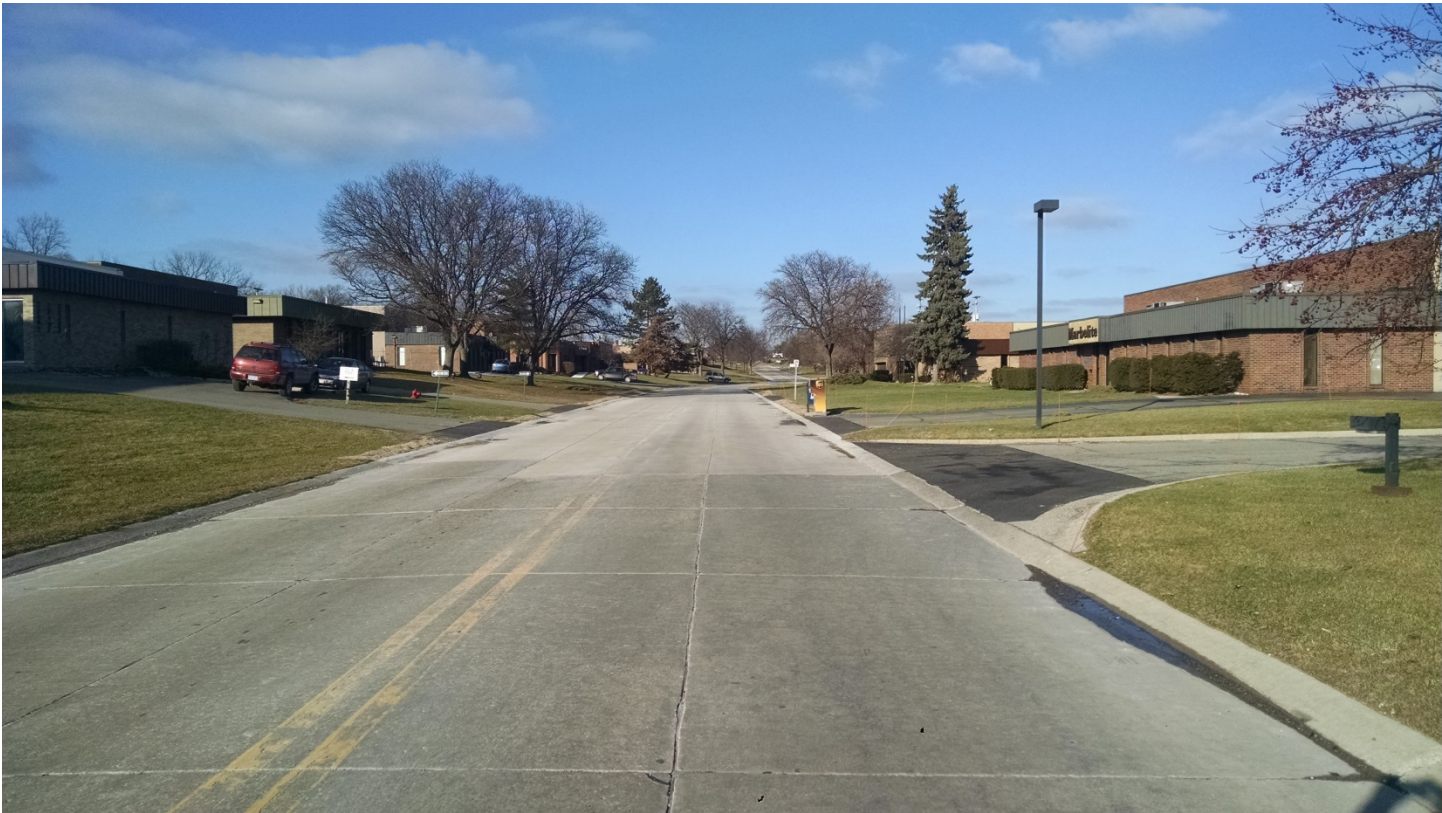
Heslip Drive – Looking north from 9 Mile
