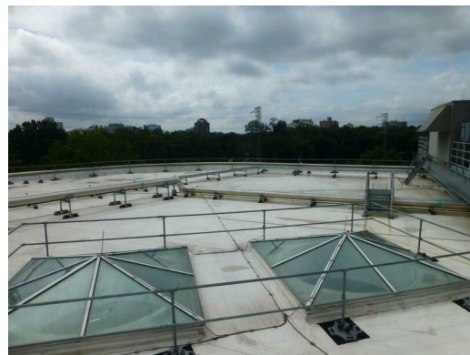
Rooftop at Bldg 1
