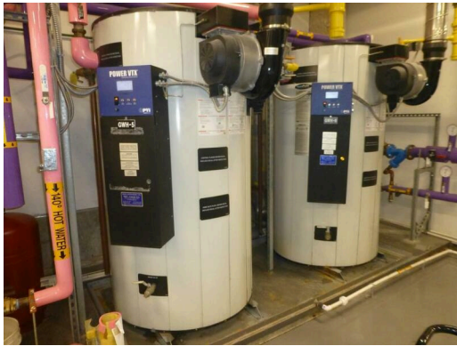
Domestic Water Heater for LAB Areas
