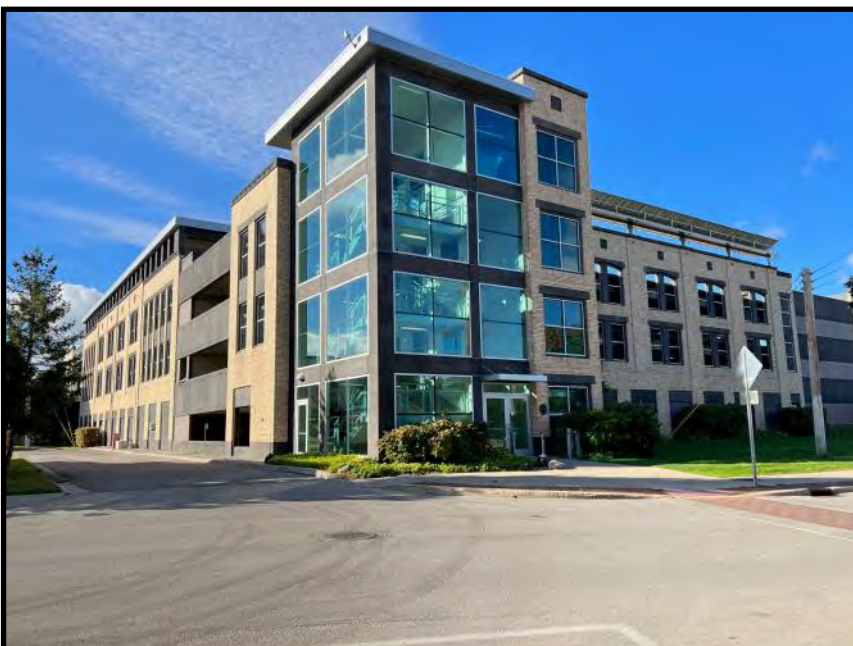
Figure E26: Parking structure in Traverse City
